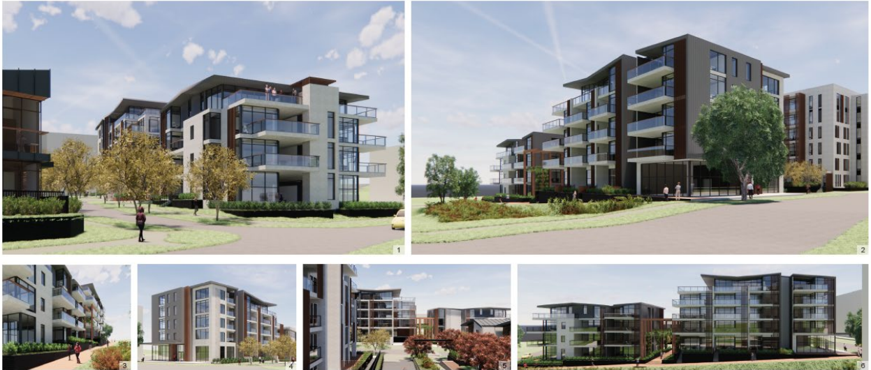
Image 2: 41-57 Fred Taylor Drive, Westgate: Four storey apartment building broken down into smaller elements/modules that step down the slope. The building presents a well-articulated and modelled mass to the street including recesses, projections and generous depth to the balconies and façade surfaces.
