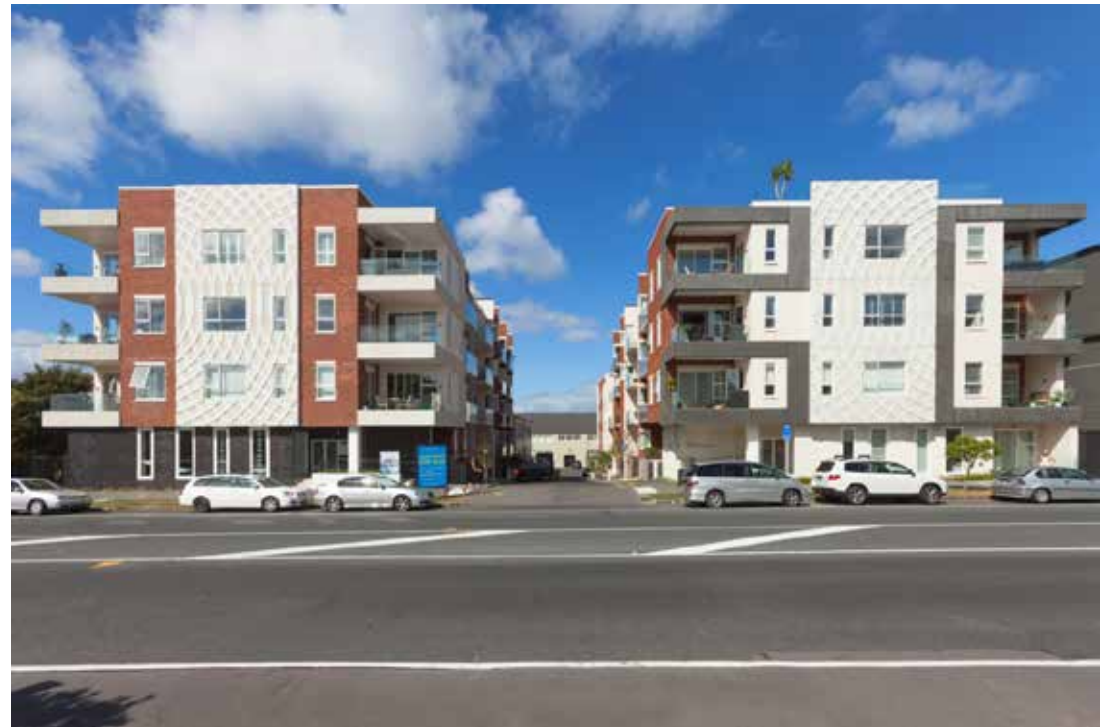
Looking towards the overall development from Surrey Crescent.
