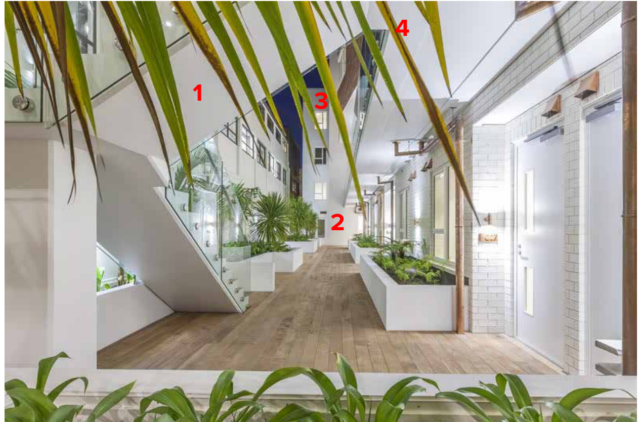
Looking into the internal courtyard which opens out on individual units on the second floor.
