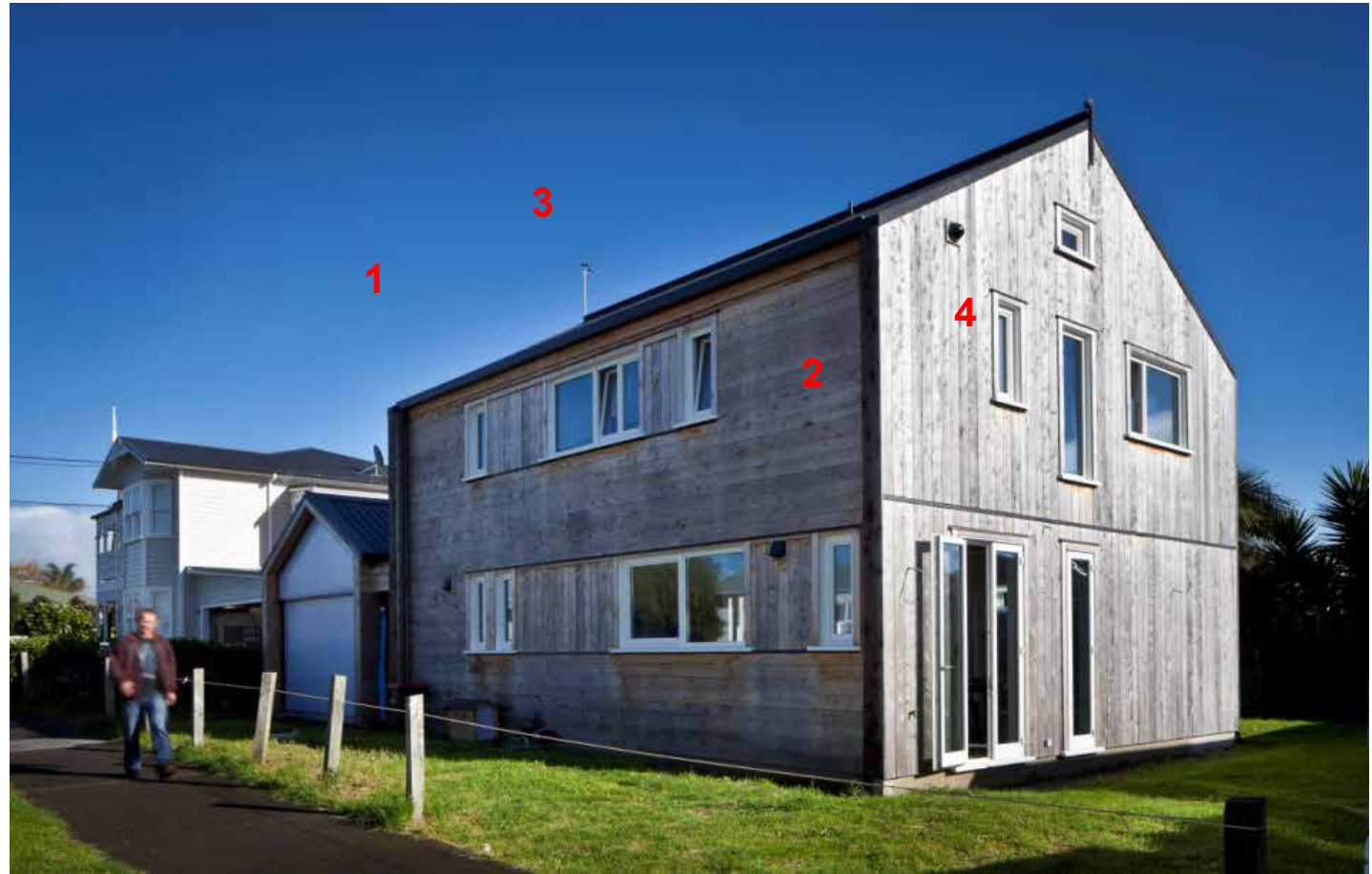
Looking towards the south-west elevation of the house from Tui Street.
