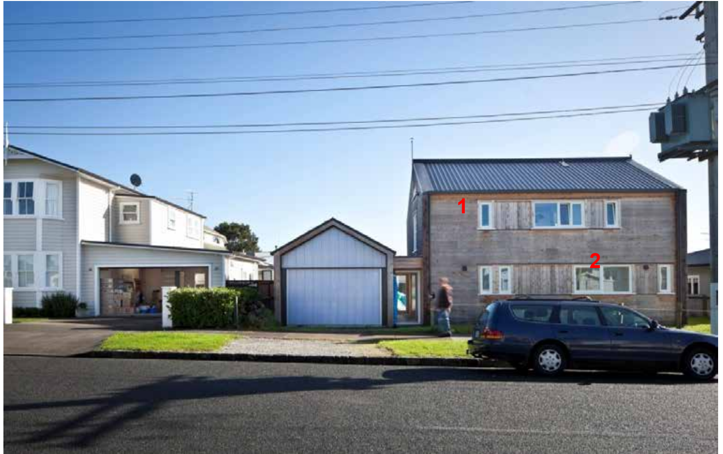
Looking towards the south elevation of the house from Tui Street.
