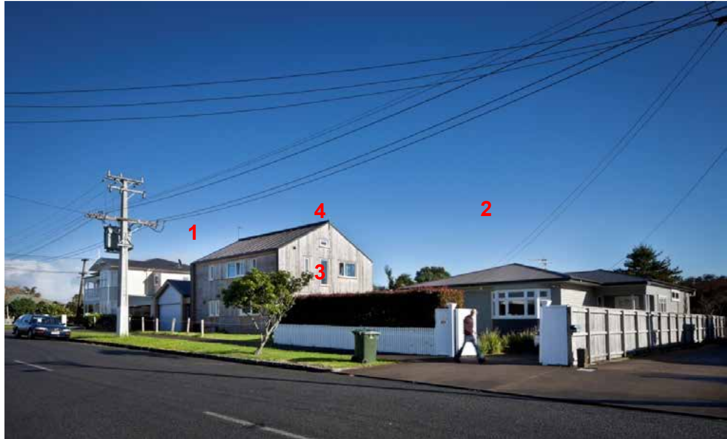
Looking towards the eastern elevation of the house from the bottom of Tui Street.
