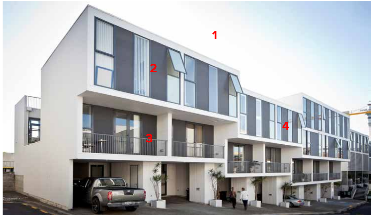
Looking at a staggered dual aspect apartment block towards the northern end of the development on Fisher-Point Drive.
