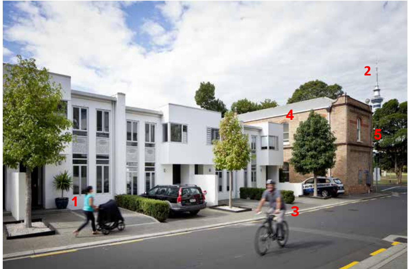
Looking towards the southern entry point of the development overlooking Victoria Park and Beaumont Street.
