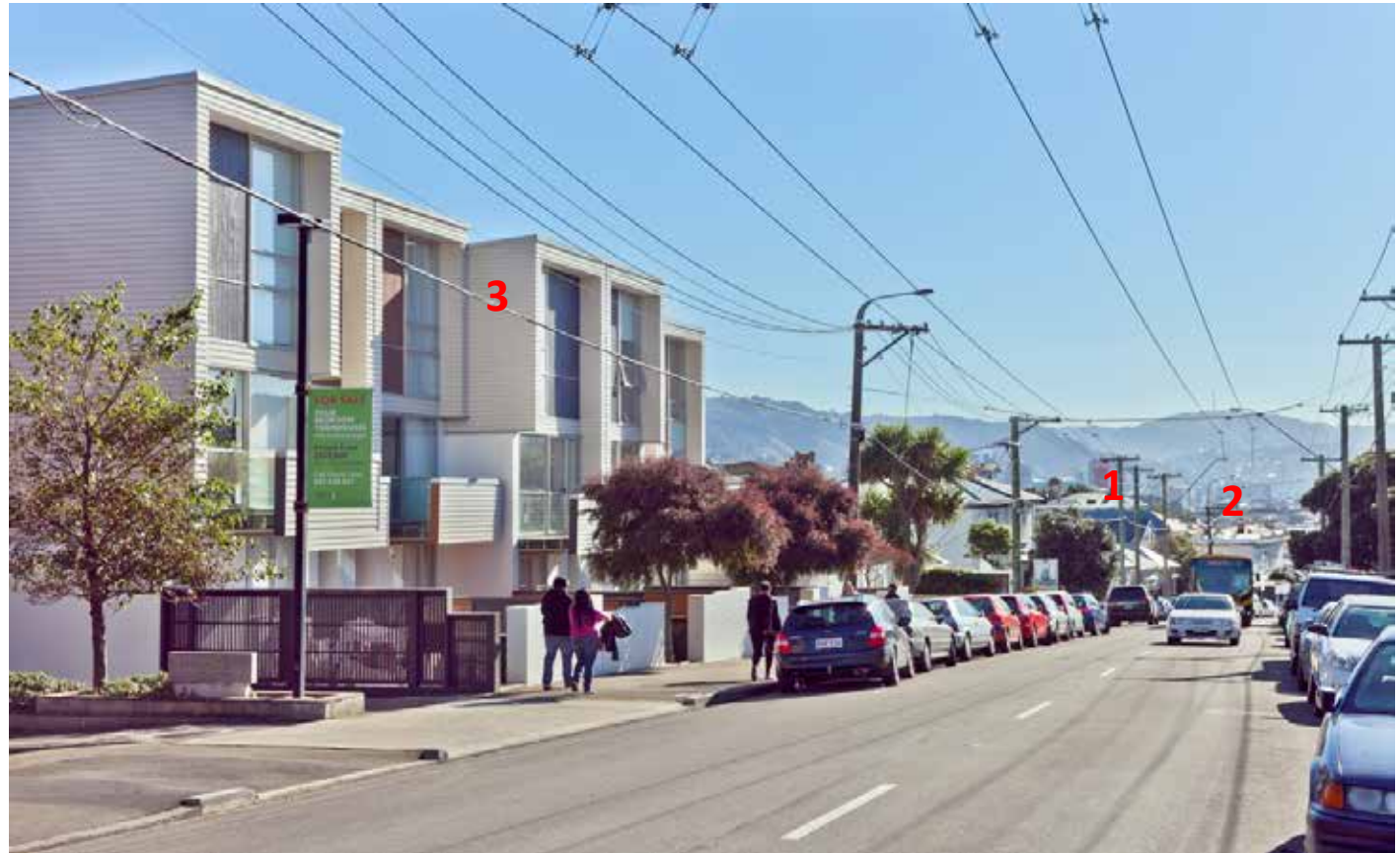
This development was on a brown-field site previously adjacent to what was Wellington's icon Athletic Park. Rintoul Street is an important north-south street that runs along the flanks of the Newtown valley.
