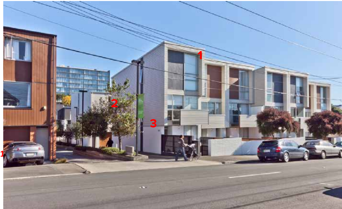
Looking towards the main entrance to the Altair complex from Rintoul Street.
