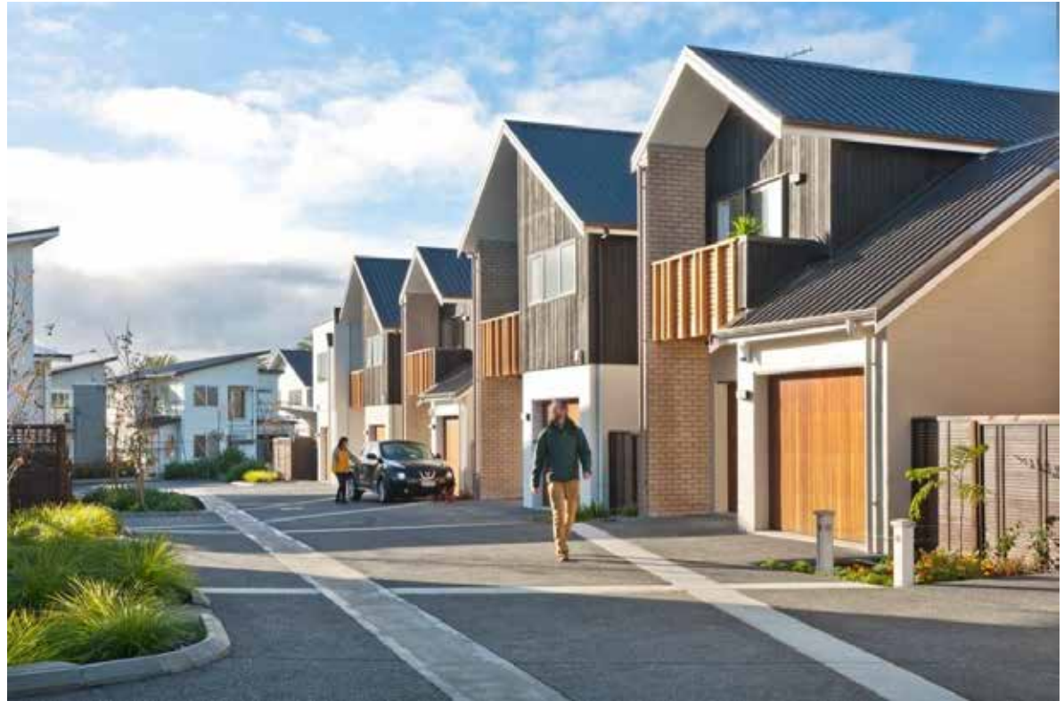
While providing an excellent edge towards Buckley Avenue, the terraces provide an attractive interface with its rear lane when viewed from Lester street.
