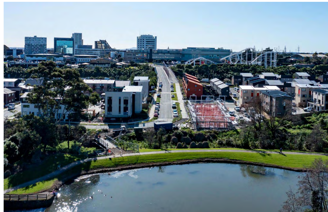
Enhanced stormwater pond and reserve in foreground; Kōtuitui terraces and courtyards and Manukau city beyond Image credit: Eke Panuku
