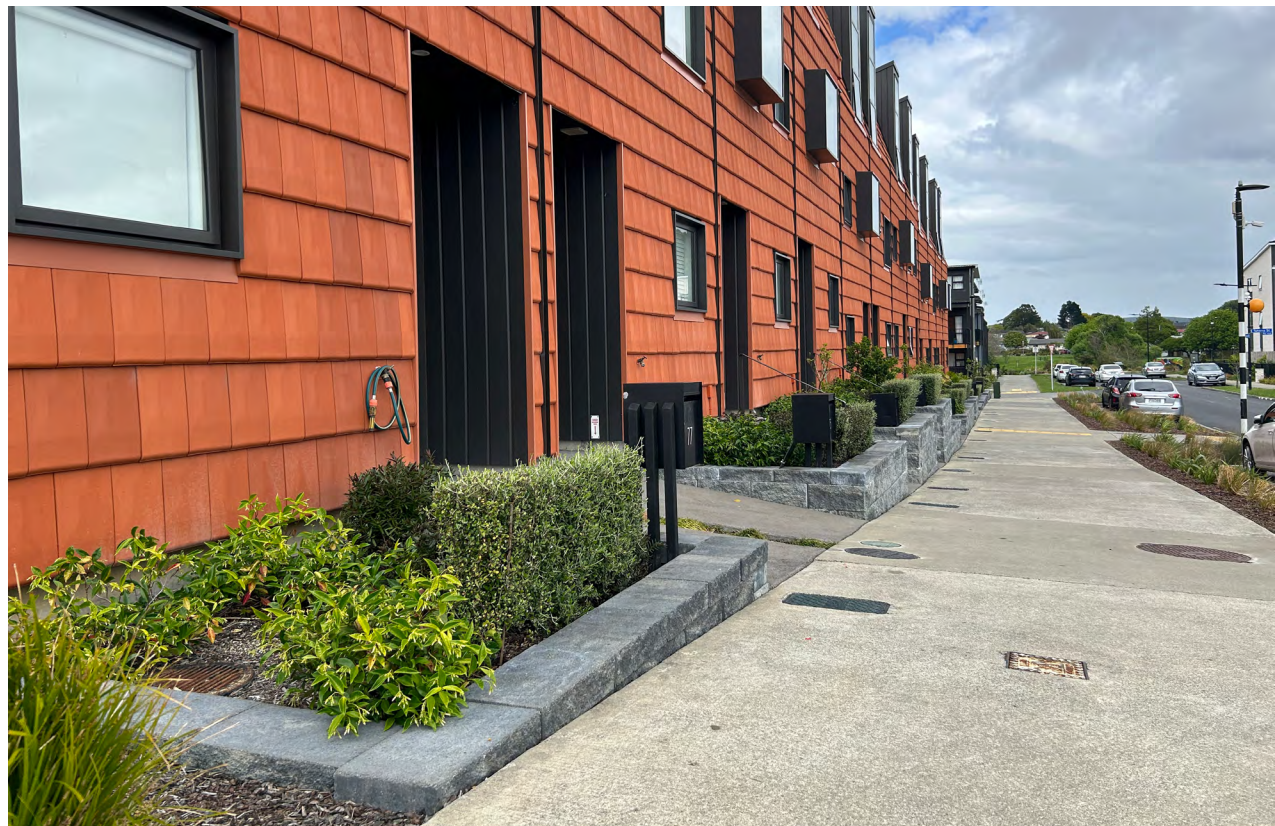
Stepped and varied blocked retaining combined with soft landscaping providing privacy and a sense of separation between public and private.
