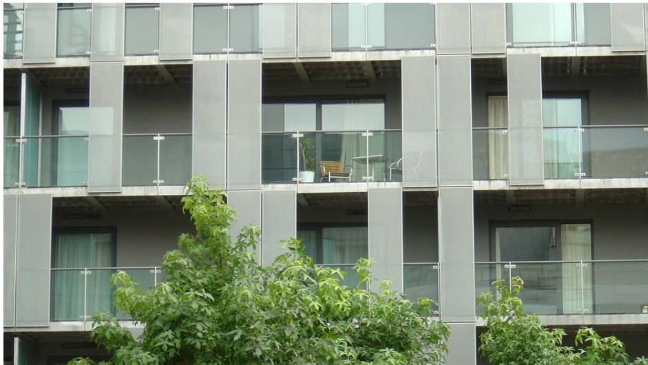
Thin mesh screens are used as part of the overall building design and provide privacy to each balcony.
