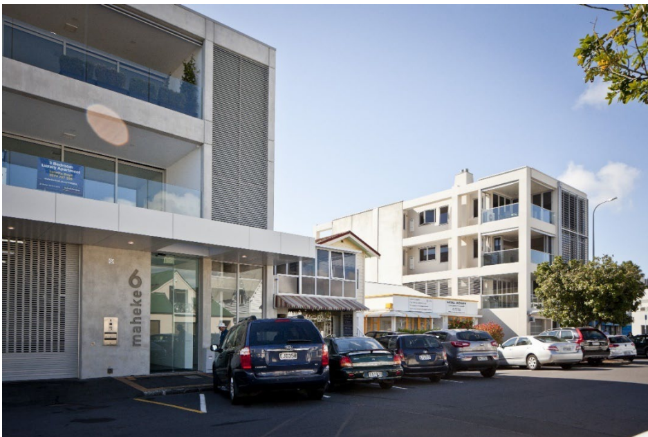
A canopy is provided to emphasise the entrance and provide shelter. Entrance is level with the street.
