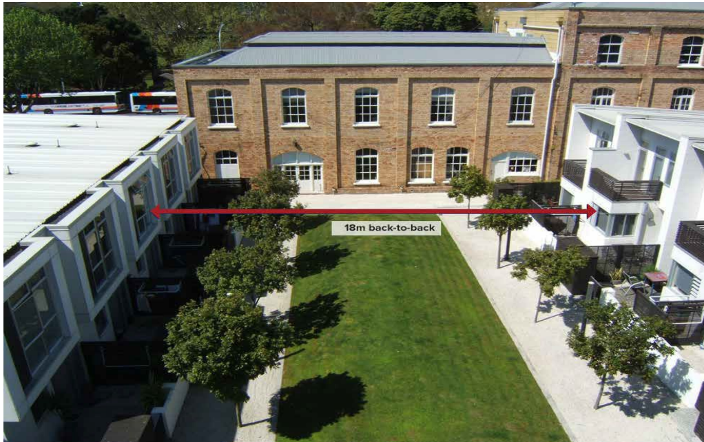
An 18m separation distance allows for sunlight access into the homes and the communal open space, as well as ensuring privacy between habitable windows and balconies.
