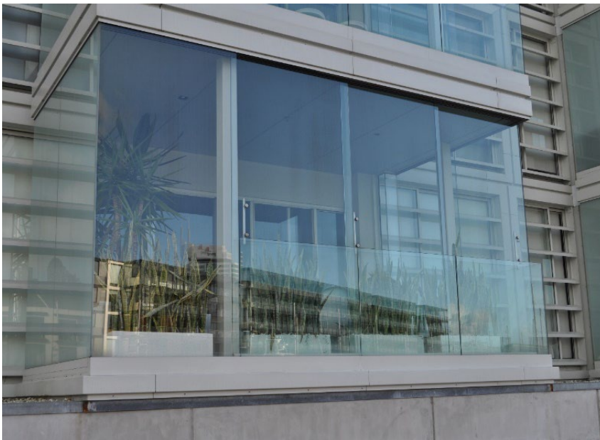
This balcony can be fully enclosed via sliding doors to further assist with noise reduction from the street.
