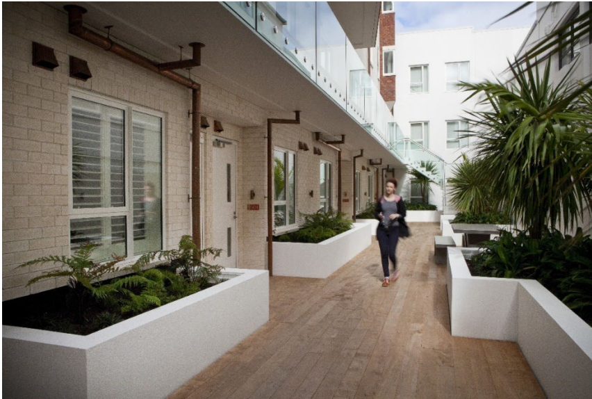
Boundary treatments provide a clear delineation between semi-public and private spaces while providing for passive surveillance.
