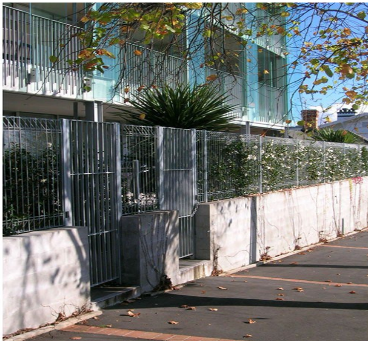
The vertical bars reduce the height of the wall and provide permeability.
