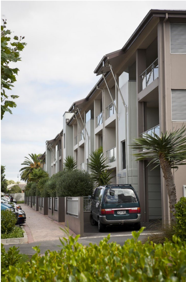
Pedestrian access is provided directly from the street.
