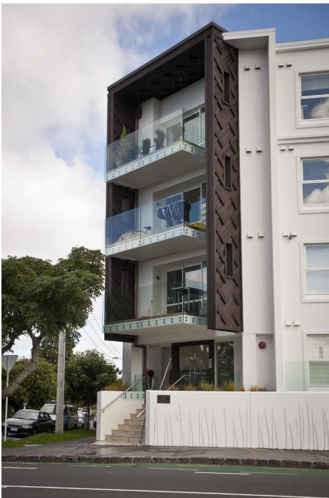
Balconies provide casual surveillance over the building entrance.
