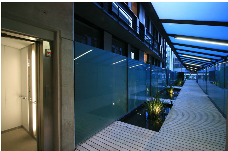
This building provides well-lit and weather-protected horizontal, semi-external access to individual apartments.
