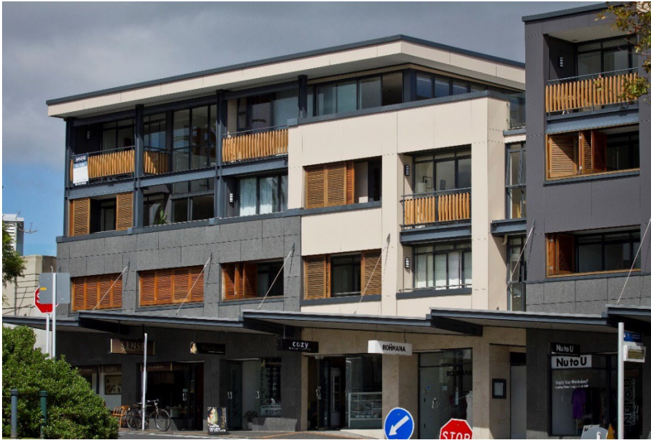
The building is designed to allow residents to adjust natural lighting to suit their needs.
