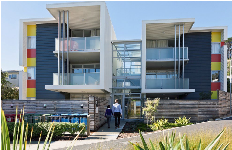
The glazed stairwell of this building separates the two halves of this apartment building – this means this entrance and circulation space are clearly seen from the street.
