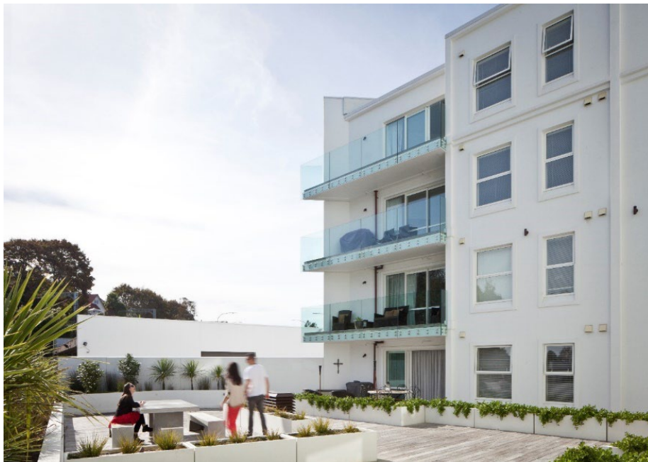
The private communal space has been designed to be well overlooked by adjacent apartments.
