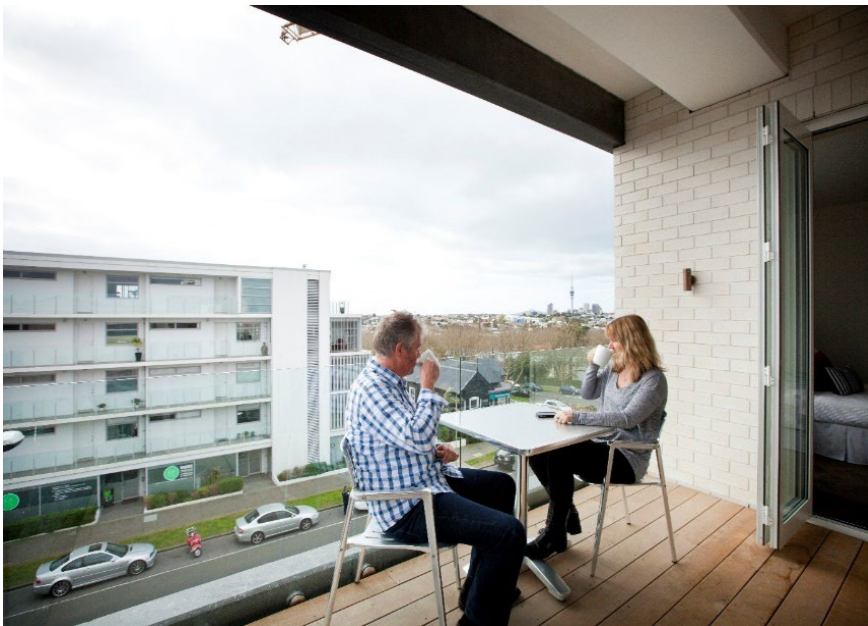
This recessed balcony offers good shading and weather protection while still being outside.
