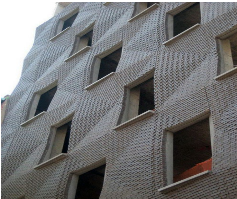
This building uses a simple material (brick) but it is used in an innovative manner to add shadow and depth to the façade.
