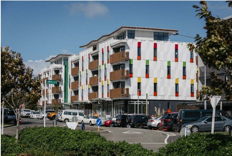
Balconies and terraces are integrated into the overall architectural form and detail of the building.
