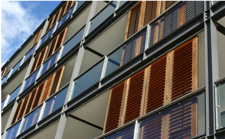
Wooden louvres are set behind the edge of the balcony, allowing them to be folded back and hidden when not needed.
