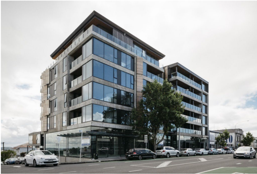
The retail premises on the ground floor means that this apartment building has a zero setback from the street.
