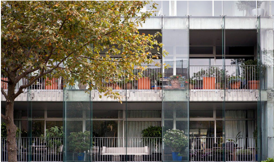
The living spaces are recessed but the balconies allow uninterrupted views of the street below.
