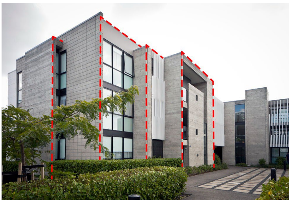
This building has been designed with a large block broken up into smaller secondary, and predominantly vertical elements to reduce the overall scale.
