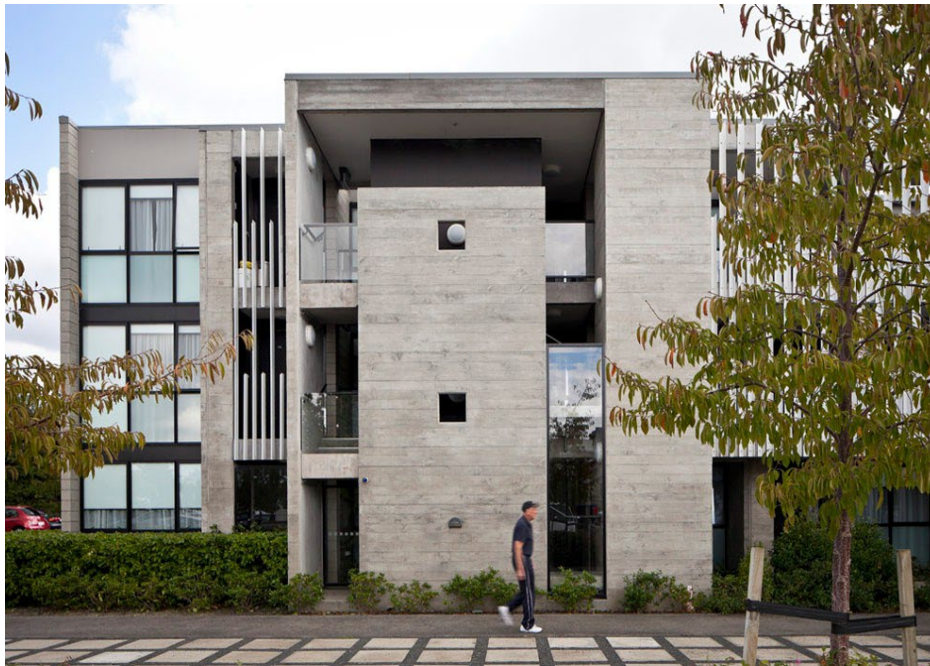
The external stairs are integrated into the overall building design.
