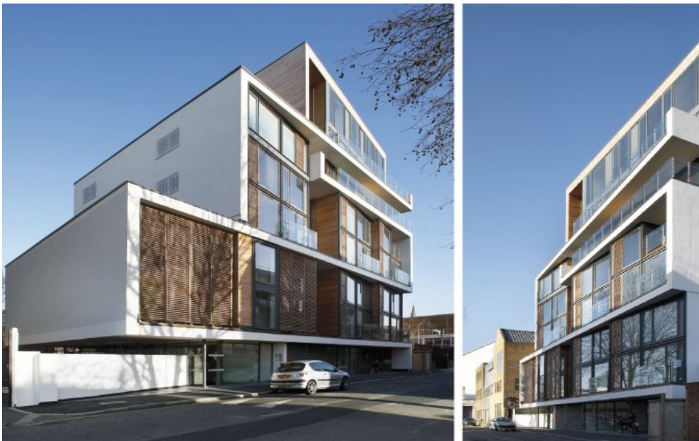
Stepping building volumes assists this building in related well to its lower-height neighbours.
