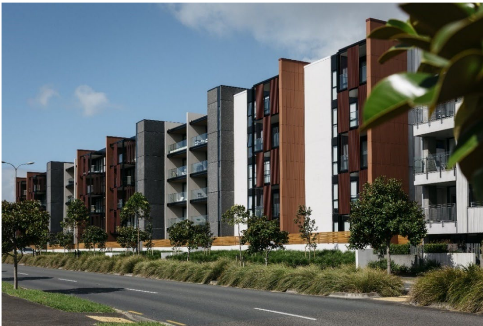
Vertical elements are well utilised to create interest on an otherwise long apartment building.
