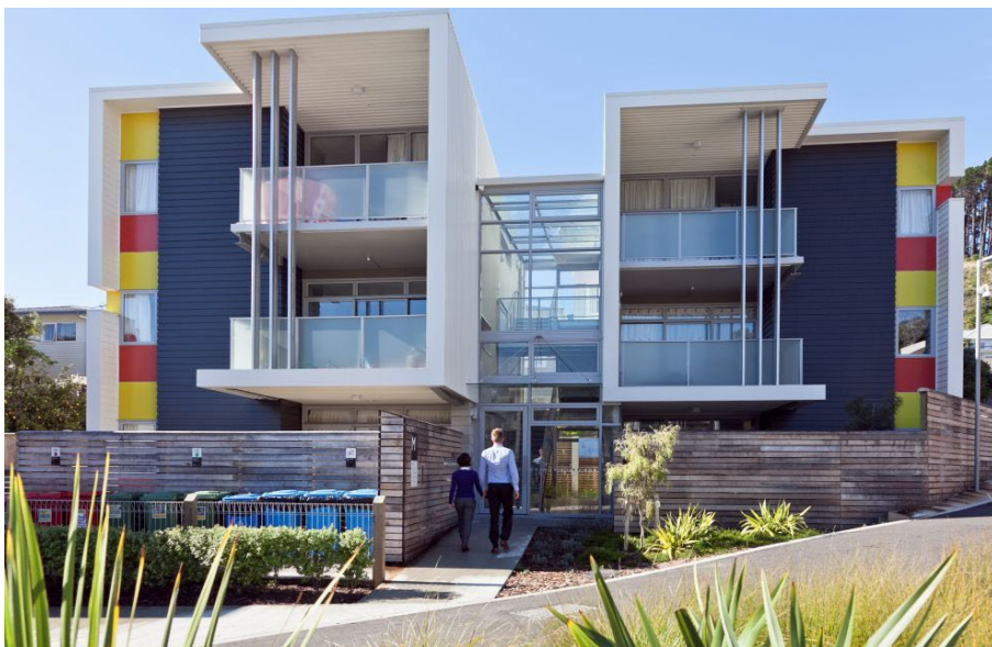
The expression of different internal functions assists in breaking down a larger built form.
