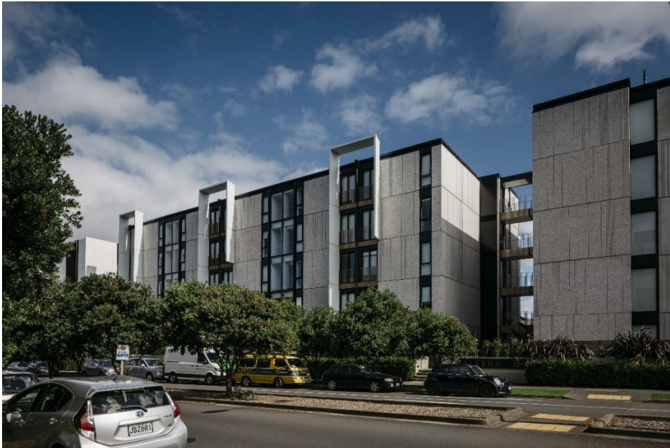
Access is by an internal, double-loaded corridor with apartment accessed off both sides of the corridor.
