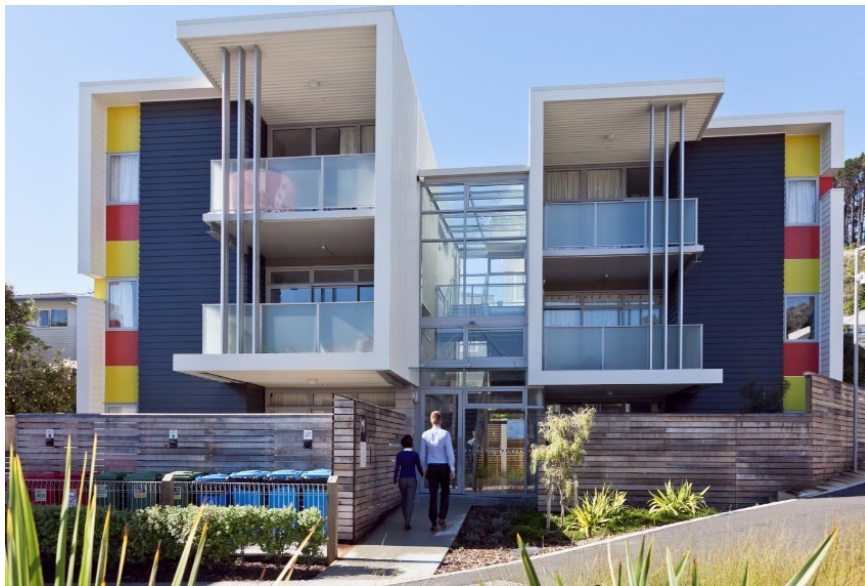
Although the bin store is at the front of the apartments it has been designed to be screened by the hedges once they mature.
