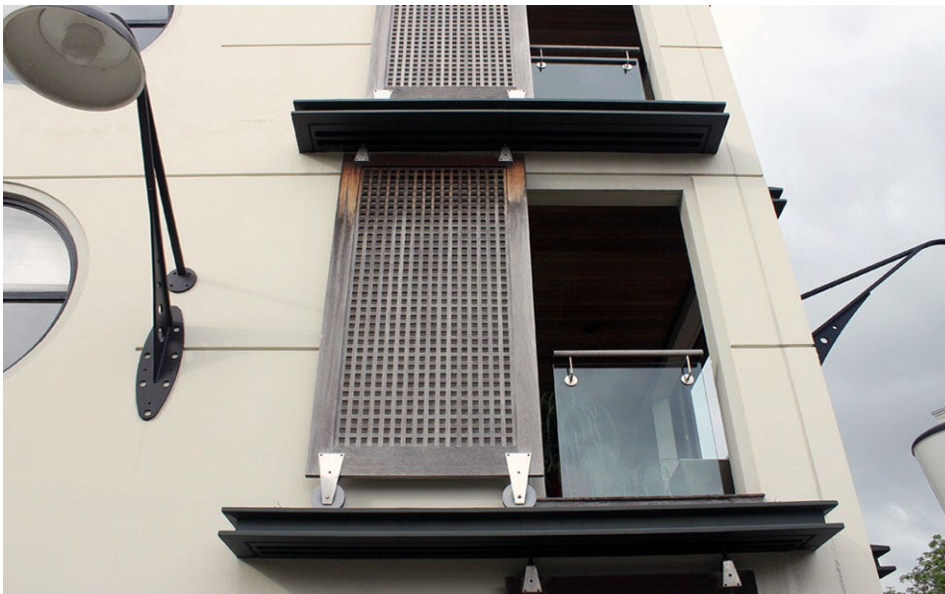
These sliding movable screens create an attractive point of interest for the building façade.
