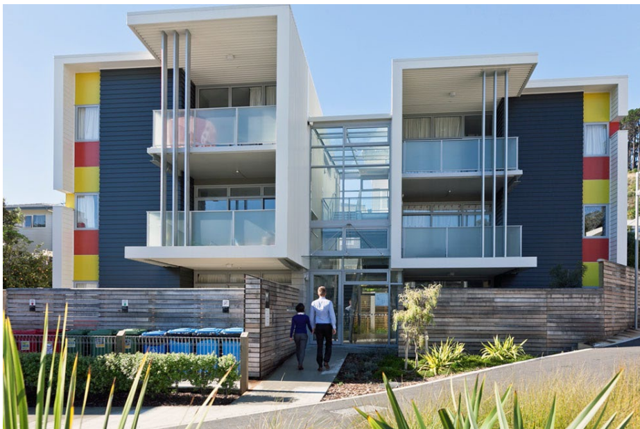
Balconies are integrated into the building to provide privacy for adjoining residents.
