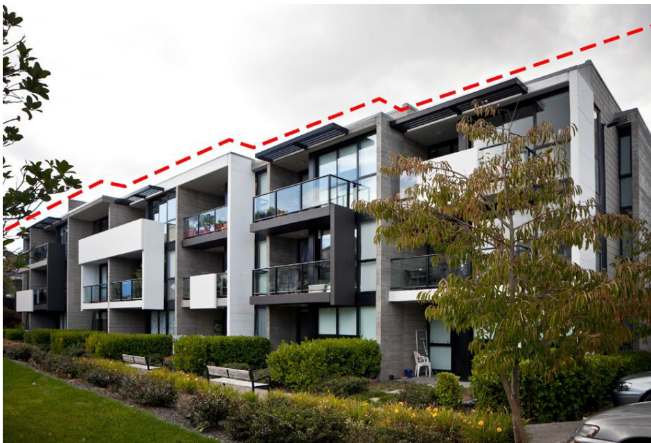
The roof form is stepped to break up the overall form and present a positive face to nearby development.
