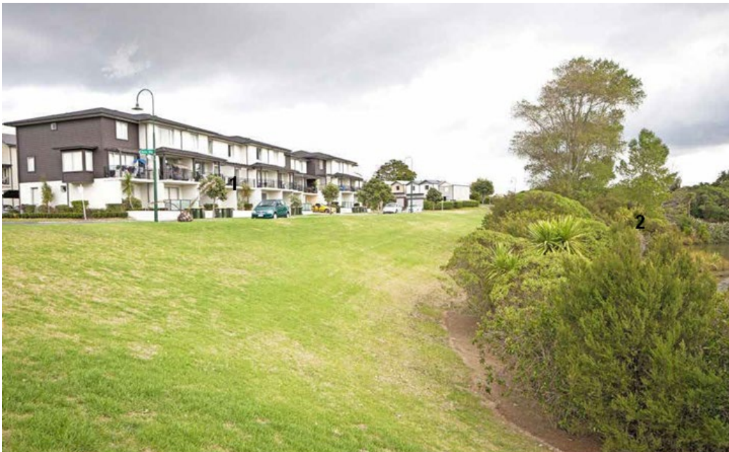
Setback distances from riparian edges protect biodiversity corridors and houses from possible flooding and establish a recreational green connection.
