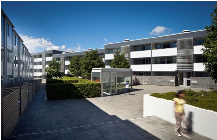
The slope of the land is accommodated within the development by a series of staggered platforms within the courtyard area.
