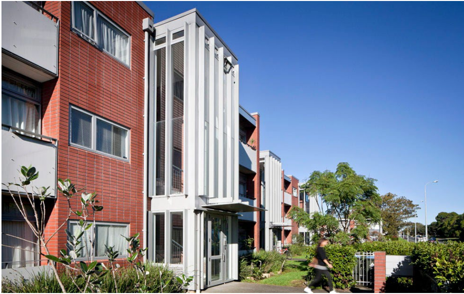
The stair cores and living areas project out from the main floor plates to break up the mass of the building.
