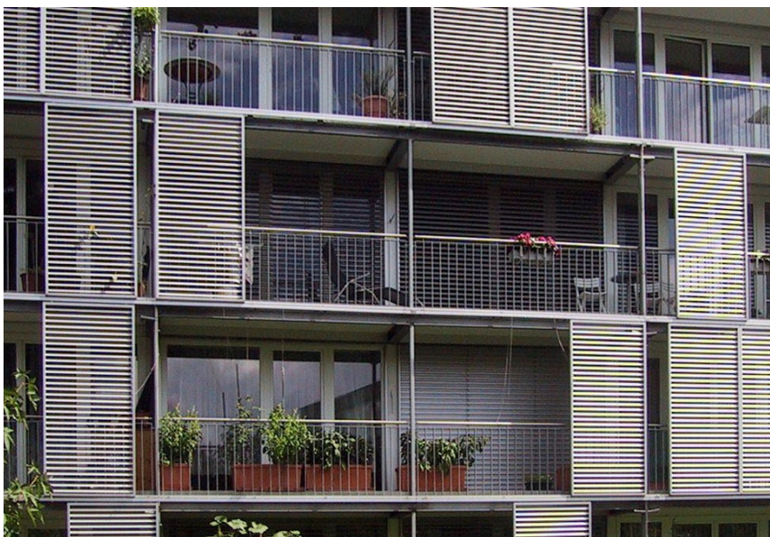
The sliding external screens can be moved by the residents as they need privacy.
