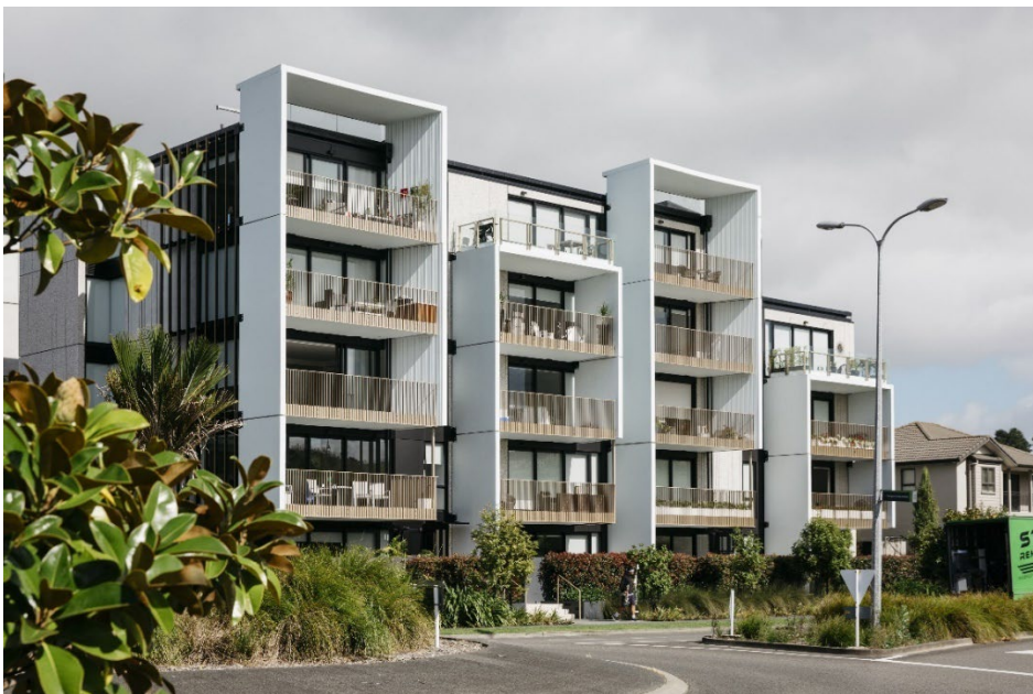
Vertical elements help to visually balance the overall size of a wide building.
