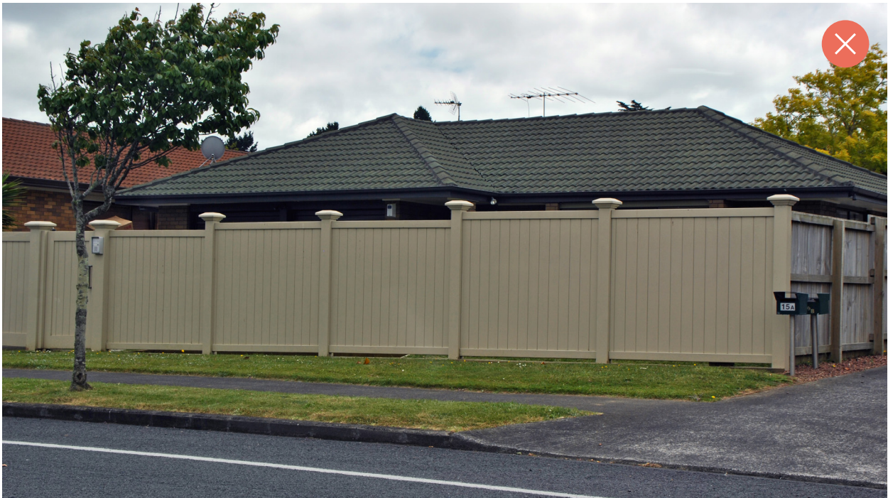
Fences over 1.4m high obstruct views into and out of the site and create a blank edge to the street. This removes an opportunity for passive surveillance and creates an unpleasant street environment.
