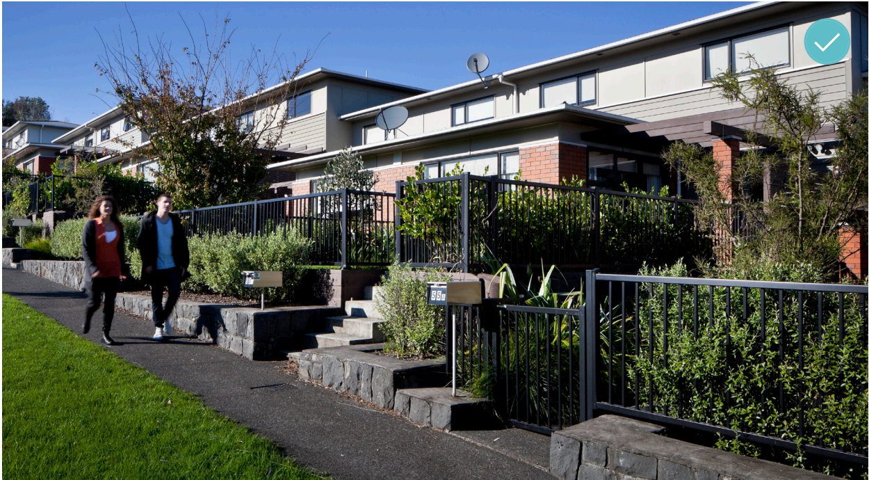
Retaining walls along the street can be enhanced with complementary fencing and planting. The impacts of this retaining wall are further reduced by stepping the walls up the slope.
