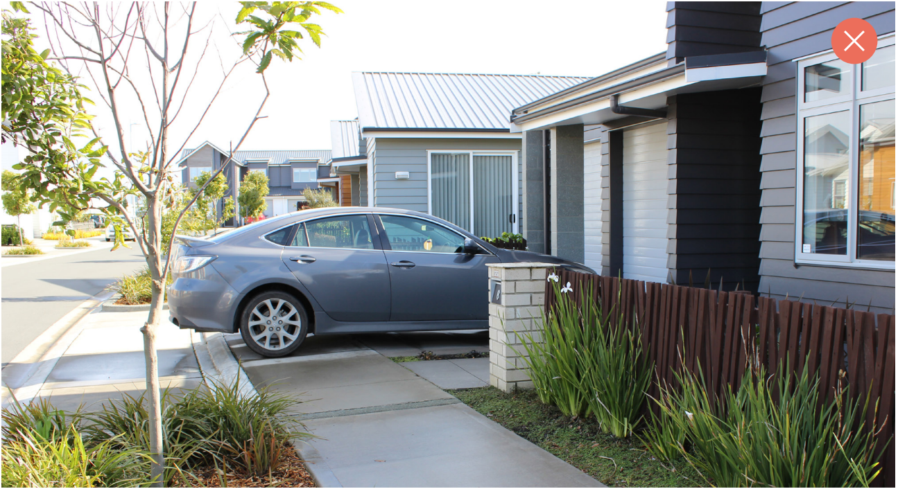
This garage is not set back sufficiently from the front boundary to allow space for a car to park in front of the garage. This results in the vehicle overhanging the footpath, obstructing the safe and easy passage of pedestrians.
