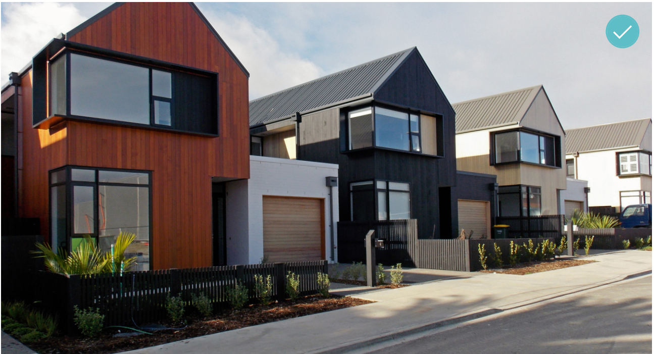
When garage makes up less than 50% of the width of the front elevation it allows space for street facing glazing, a front door, and an attractively landscaped front yard.
