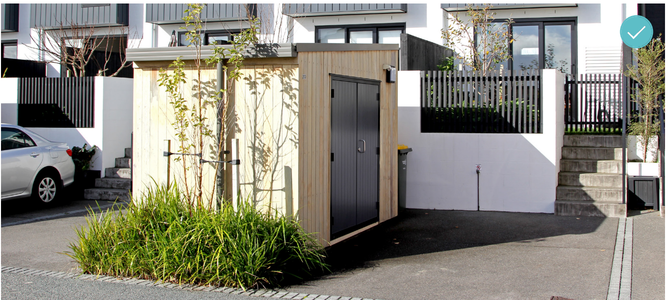
A storage shed is provided in a rear service lane. The shed is attractively designed, lockable and weather tight.
