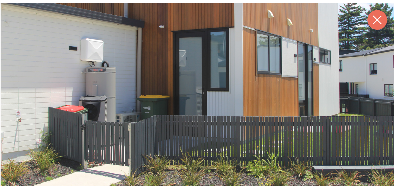
Utilities have not been integrated into the design of the site, detracting from the streetscape and what would otherwise be an attractive development .
