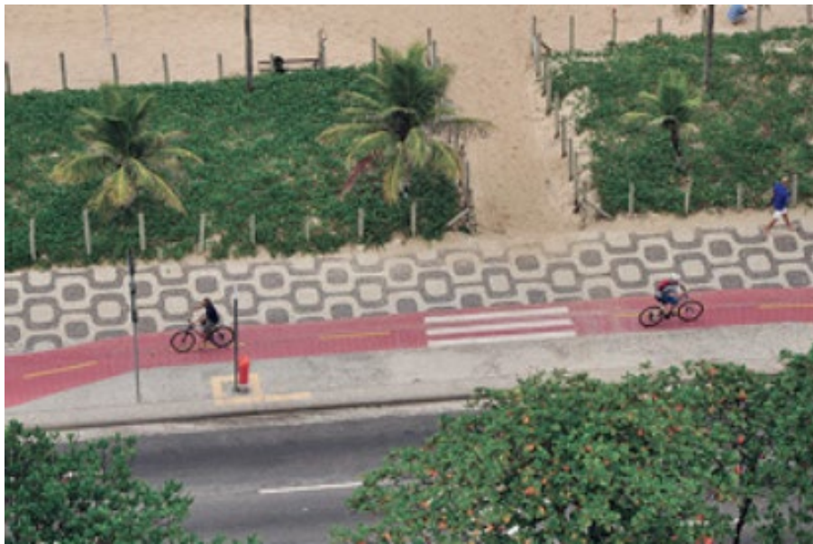
Changes in materials and colour used to clearly differentiate cycle and pedestrian routes from the carriageway
