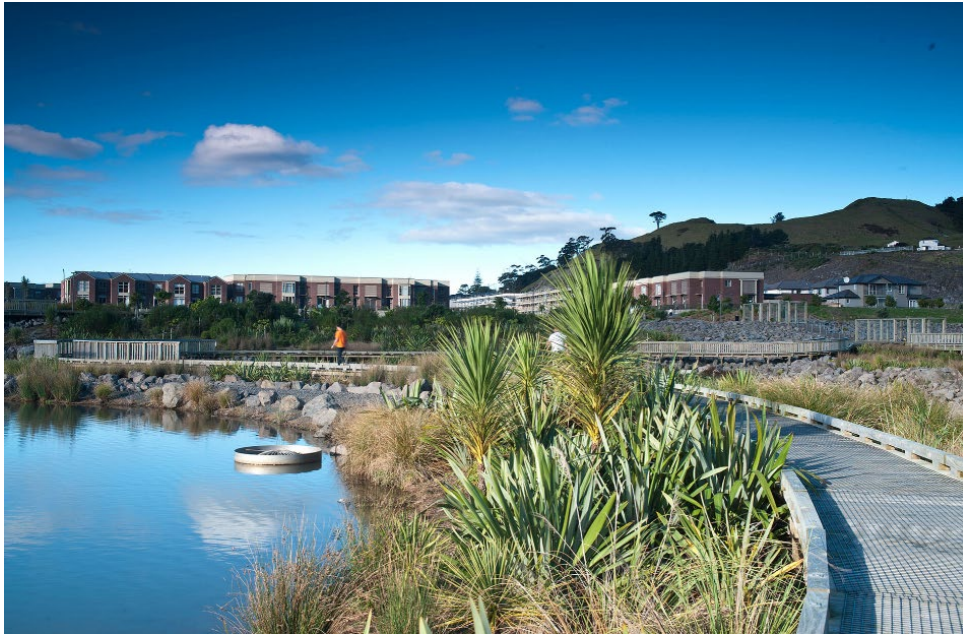
Above and below: Stormwater treatment and native planting integrated into, and a feature of the subdivision. Image credit (above): Candor3
