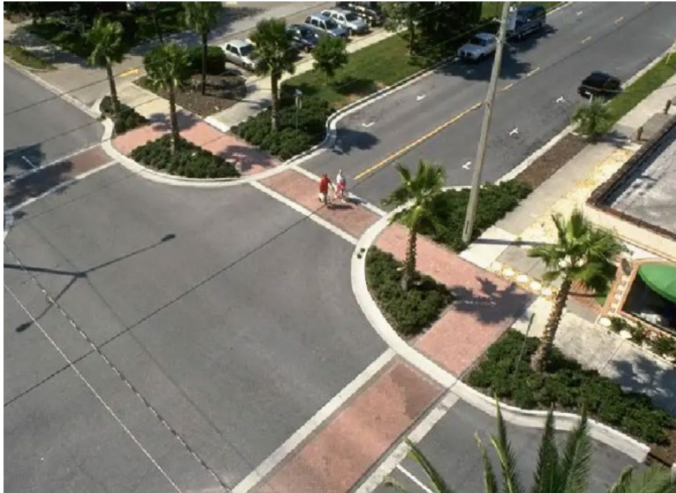
The intersection corners are enlarged and attractively enhanced while tightening the street to slow vehicles
