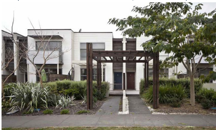
A pergola emphasises the front door.
