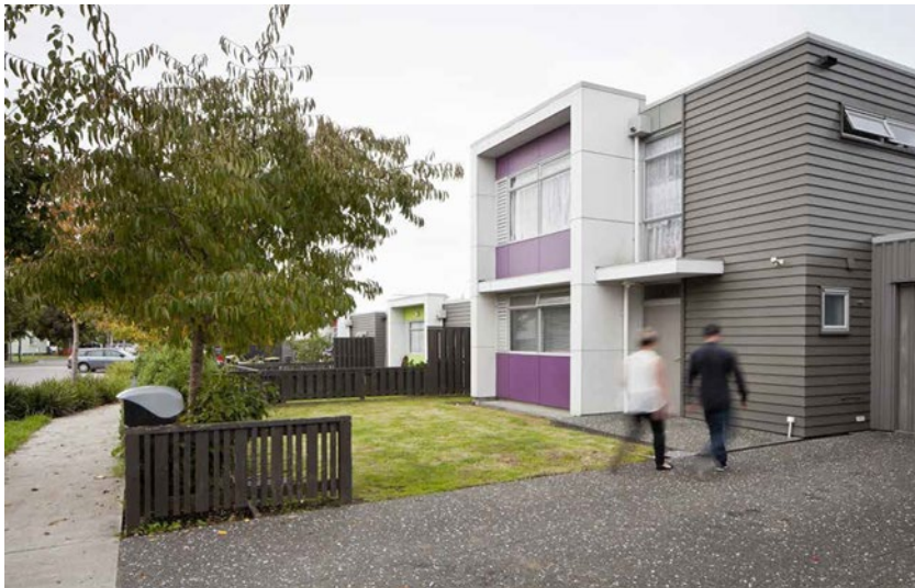
Form and colour make the active parts of the facade more prominent.
