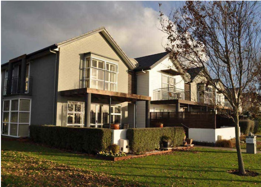
Terraced housing is orientated to make the best use of sunlight to principal living areas and private open spaces.
