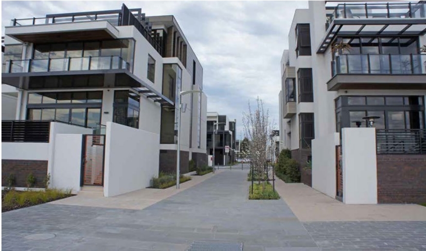
Balconies face the street and away from dwellings opposite to increase privacy.
