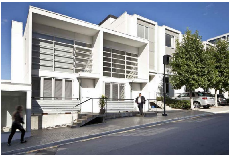
The terraced house works with the existing topography to maximise views and privacy.
