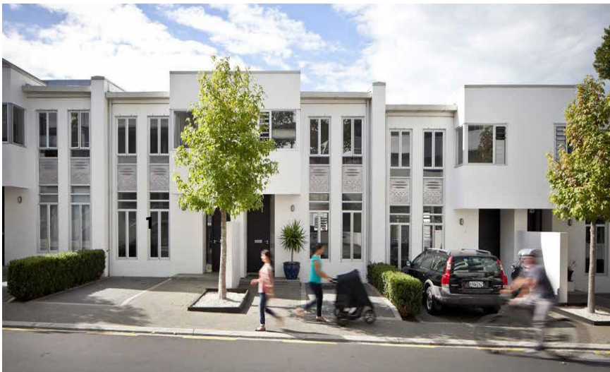
The building has many windows and front doors facing the laneway to provide passive surveillance, whilst managing privacy with narrow window sizes.
