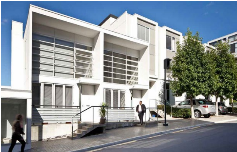
Deep recessive eaves, mechanical louvers and planting prevent overheating from the high summer sun.
