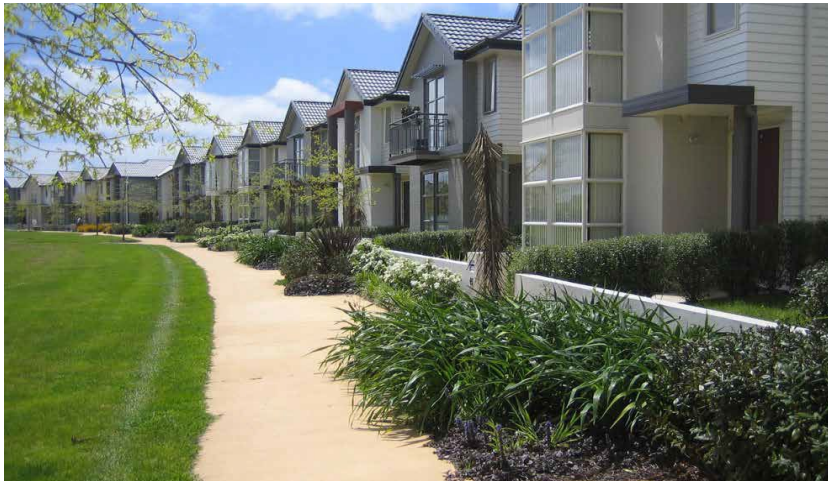
Low walls provide passive surveillance and planting softens the edge.
