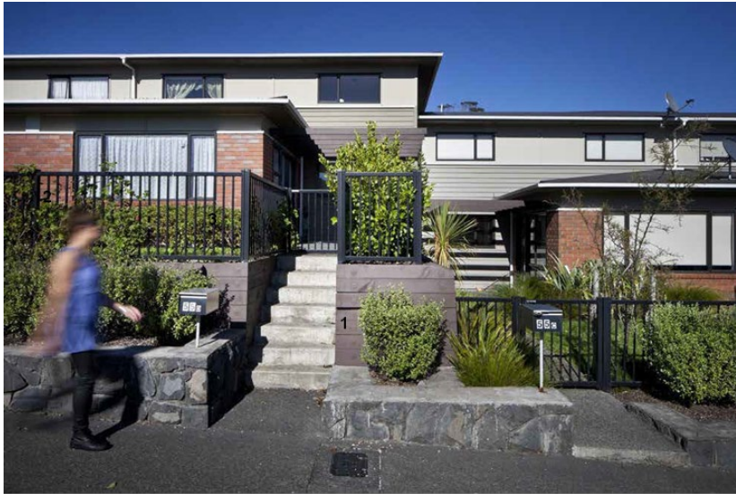
Retaining walls are stepped and landscaped, whilst permeable fences provide passive surveillance and level changes with the street offer privacy.
