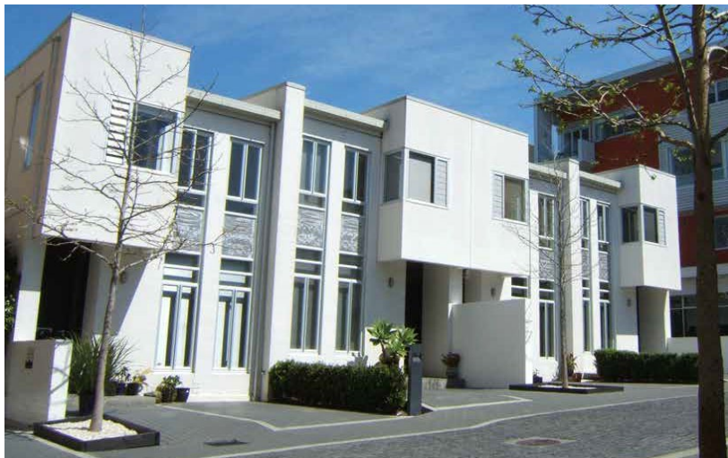
Mirroring the central units and 'handing' the outer units create a variety in building form, reducing the appearance of repetition.
