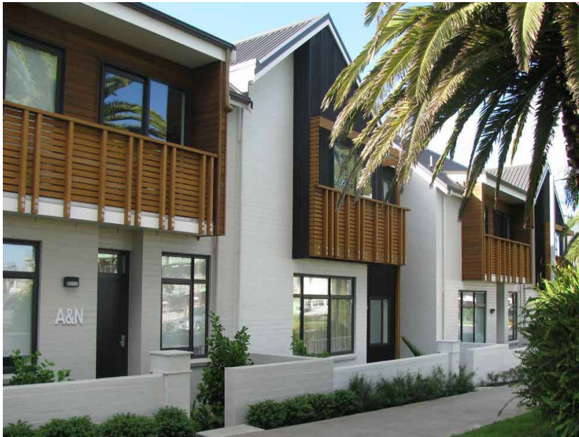
Cedar balconies create a horizontal band of contrasting colour, and add richness and texture to the street scene.
