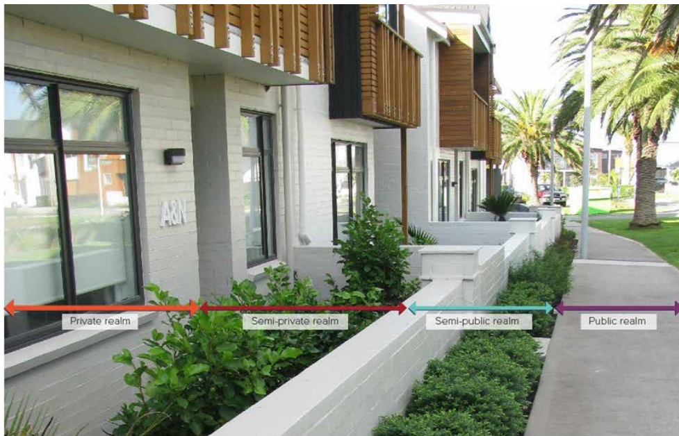
The front wall and landscape marks the boundary between the public and private realms
