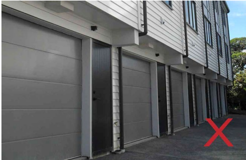
Garages dominate the accessway.
