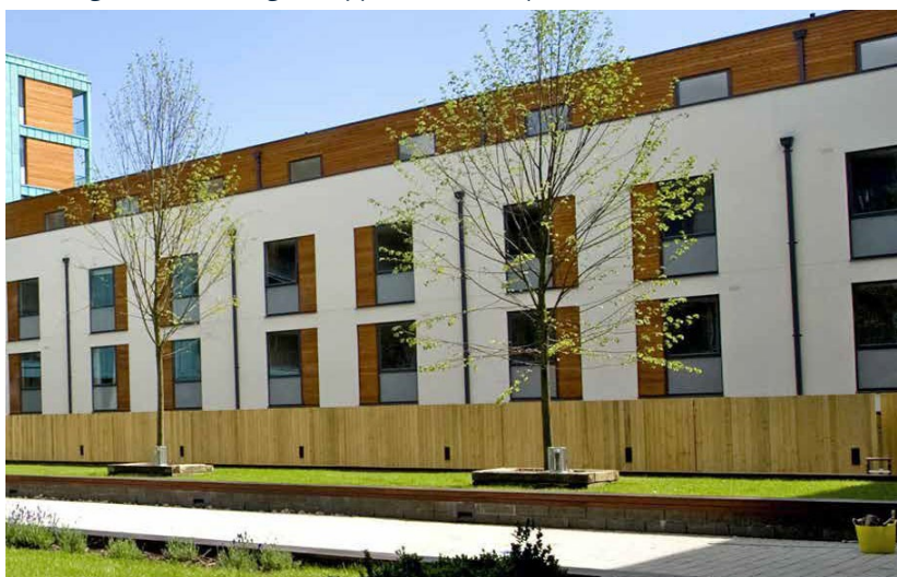
The position of windows and the downpipe of a contrasting colour establish vertical and horizontal lines, defining each dwelling within the larger building.
