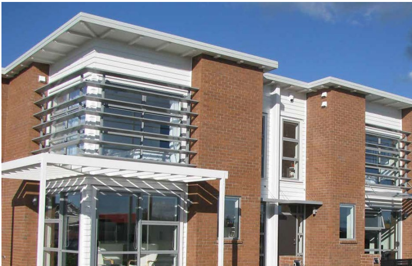
Pergolas and horizontal slats are used to provide shading in the summer.
