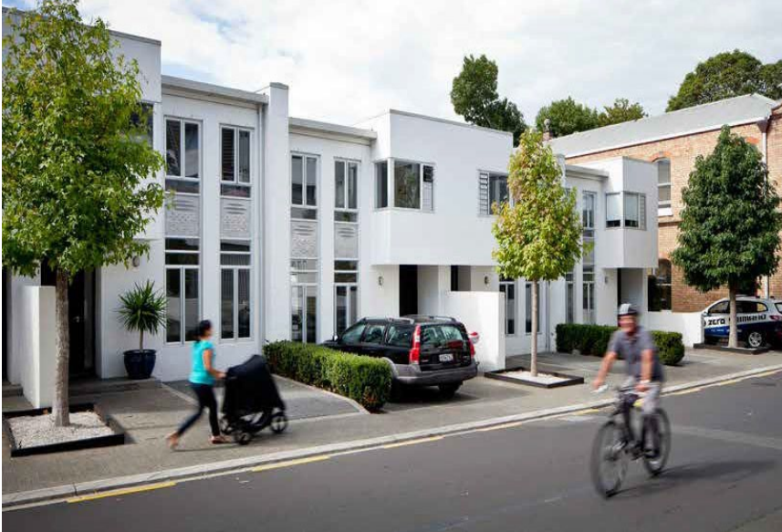
Entry porches are clearly visible from the street and the first floor extends over the ground floor entry point to provide weather protection.
