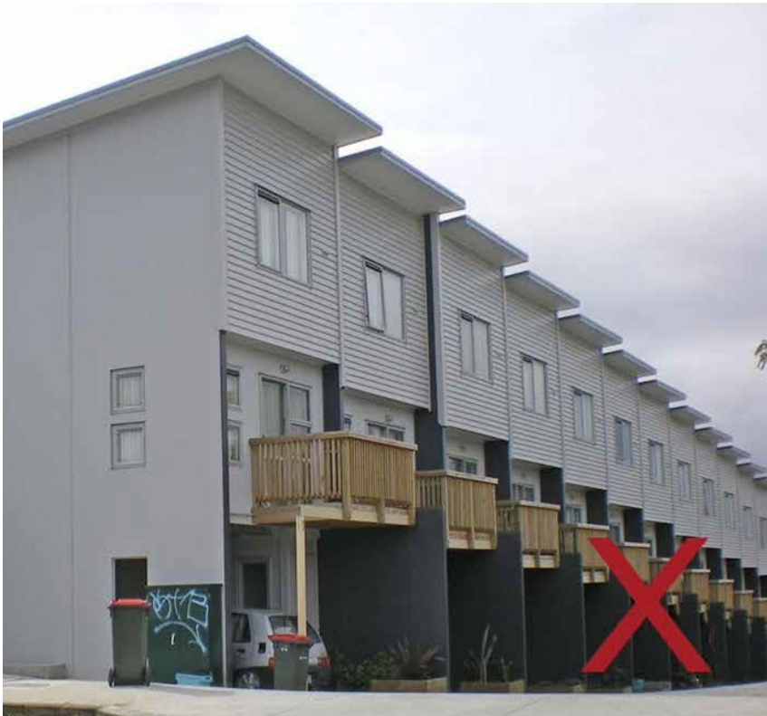
Repetitive façade design increases the scale and massing of the development and presents a poor-quality building to the street.
