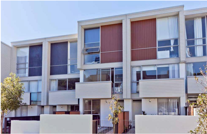
The rear elevation expresses individual aspects of individual houses / internal spaces by recessing façade elements, and using different materials and colour.
