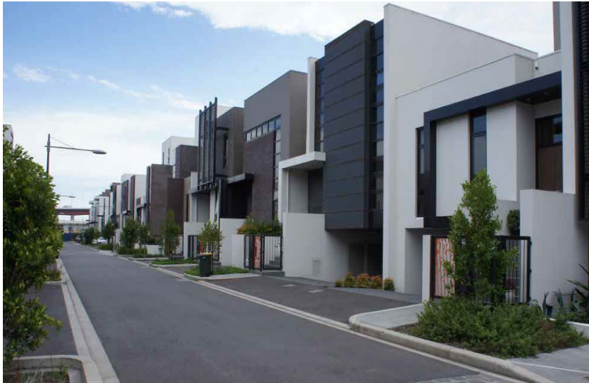
A varied but co-ordinated palette of materials establishes a sense of place.
