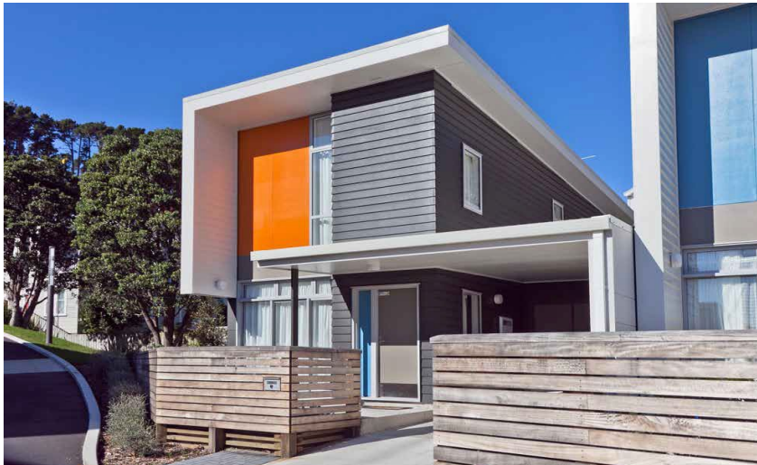
Bin stores, utility boxes, and weather protection at the entrance are integrated into the overall design.
