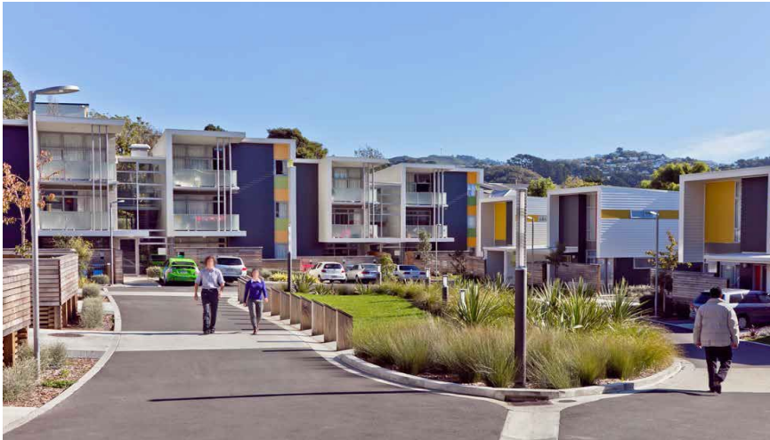
Large balconies provide a sense of overlooking and safety in the laneway and communal space. Lighting provides safety at night.
