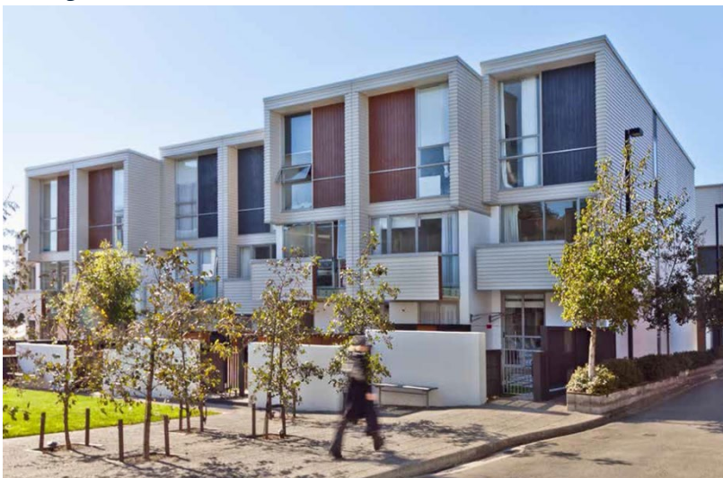
Strong vertical and horizontal lines using colour and projecting and receding building elements. Building mass is also reduced through staggering the building line and emphasising vertical elements.
