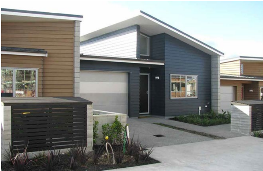
Bin storage areas are screened and integrated into the design of the fences.
