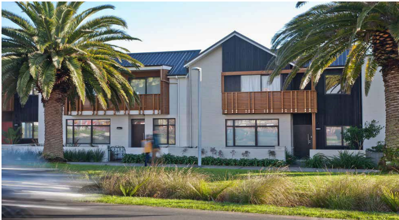
Timber decks provide delineation between the first and ground floor.
