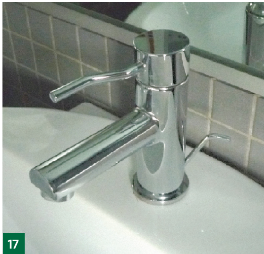
Bathroom tap mixer with lever handle. Levers make it easier for everyone to use the tap.
