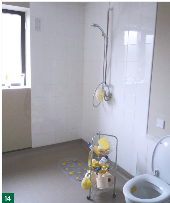
Level access showers can be fitted with doors or curtains to control the spray of water.
