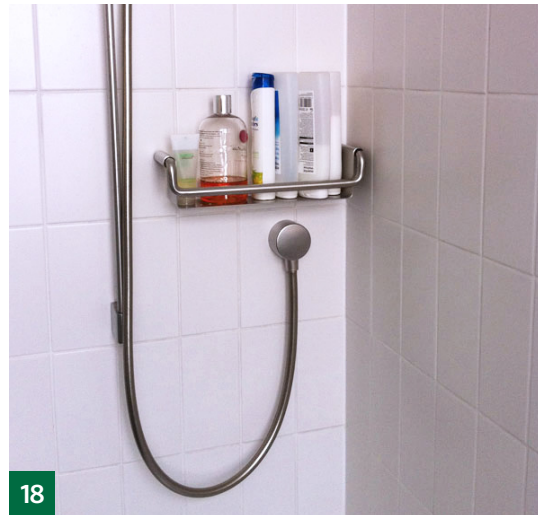
Storage for toiletries is conveniently located for use in the shower, avoiding the need to bend down or stretch across to pick up an item.
