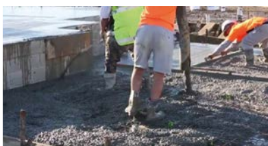
Working with concrete 2:49
