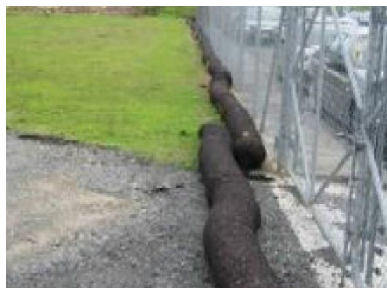
Figure 92: Silt sock with 1 m overlapping joint
