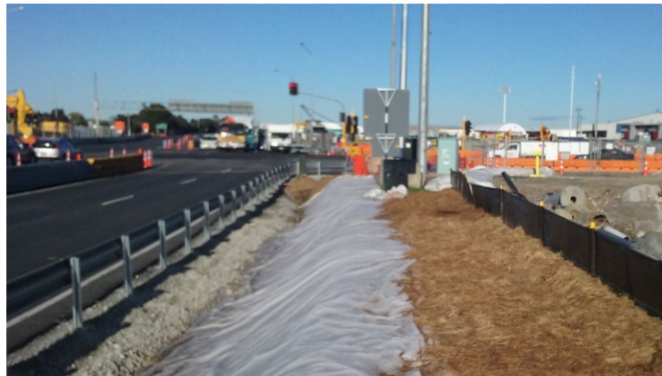
Figure 109: Progressive stabilisation in limited space
