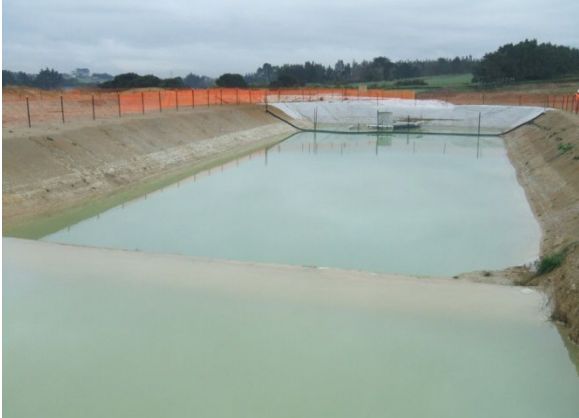
Figure 76: Level spreader across the full width of the pond
