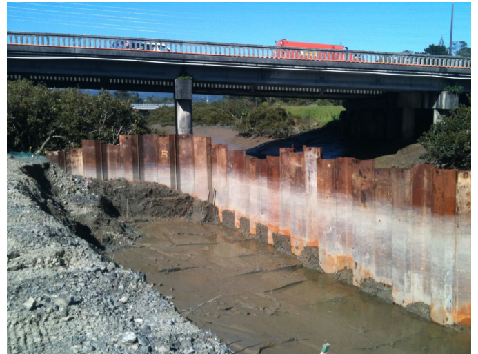
Figure 132: Sheet pile coffer dam
