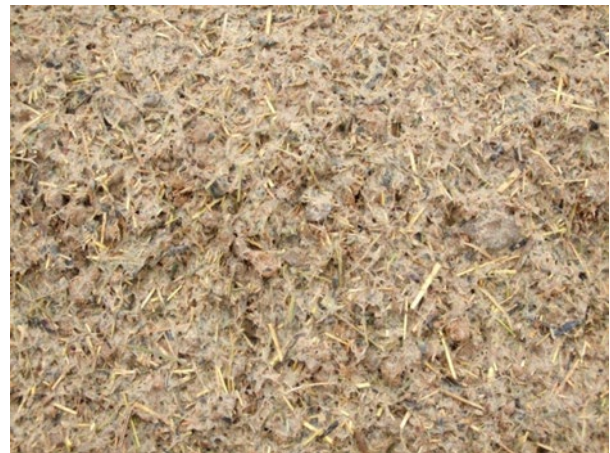
Figure 56: Hydrohay as applied
