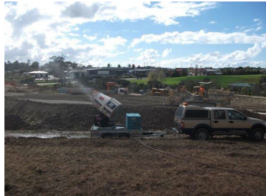
Figure 127: Snow blowing machine to provide dust control during a liming operation
