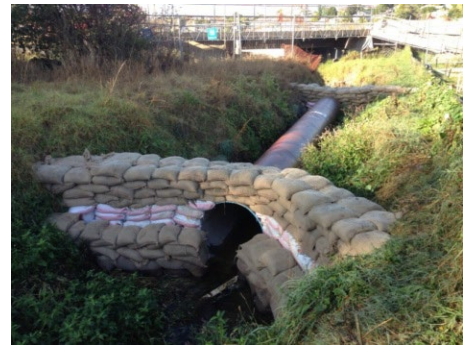
Figure 115: In the process of constructing a temporary crossing
