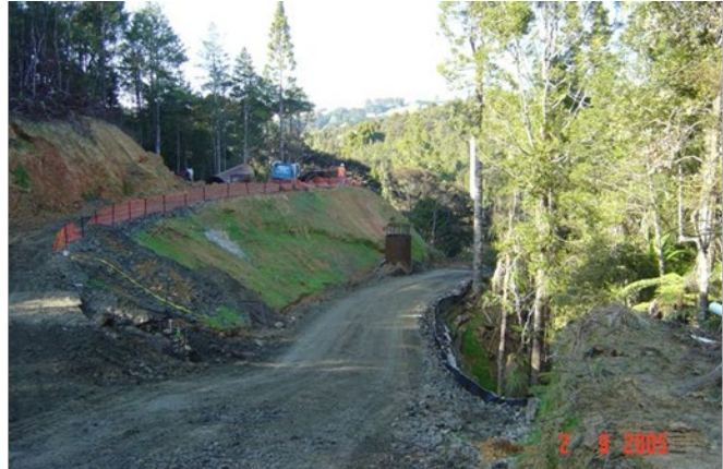
Figure 11: Northern Motorway construction site - minimising disturbance
