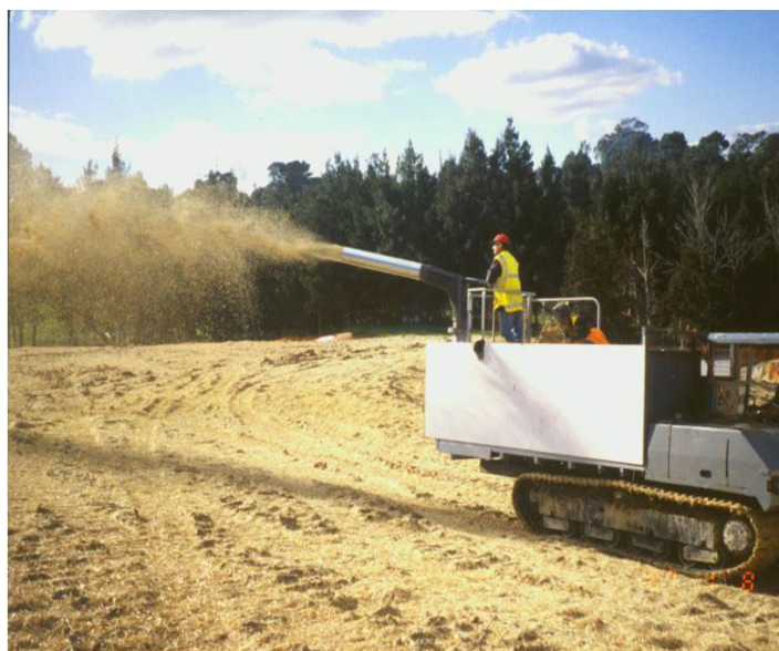
Figure 54: Specialist application of hay mulch
