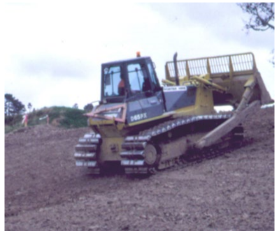
Figure 39: Surface roughening with bulldozer
