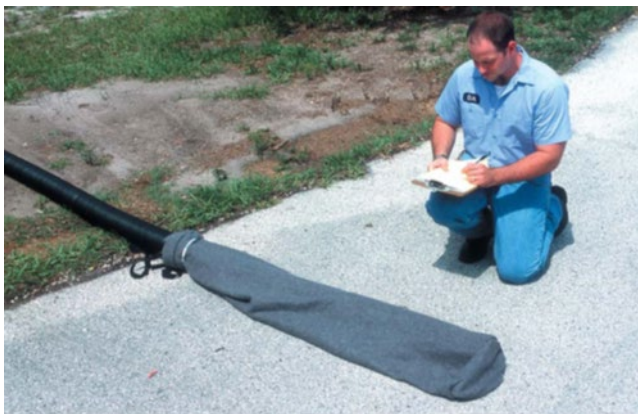
Figure 106: Dewatering bag and pipe sock
