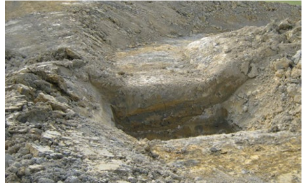
Figure 21: Drop out pit
