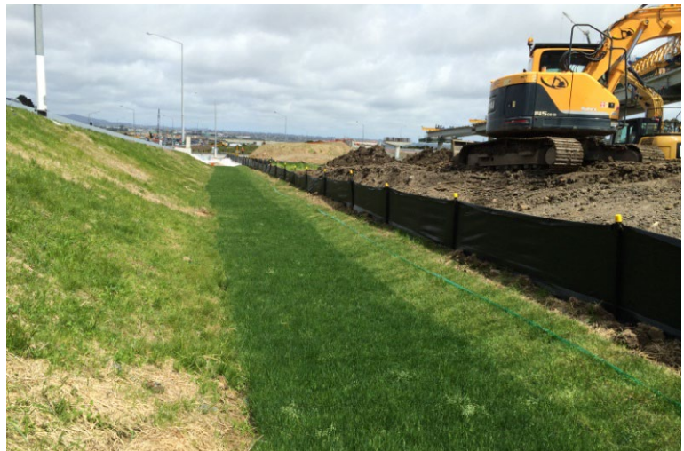
Figure 53: Turf used to provide instant stabilisation of the swale allowing for early commissioning of the device
