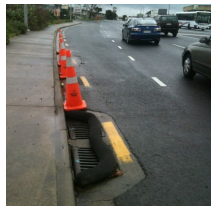
Figure 99: Installation of a silt sock to provide some protection to the catchpit
