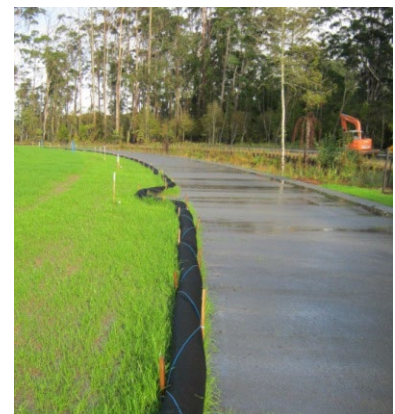
Figure 96: Silt sock used to provide control during final landscaping works
