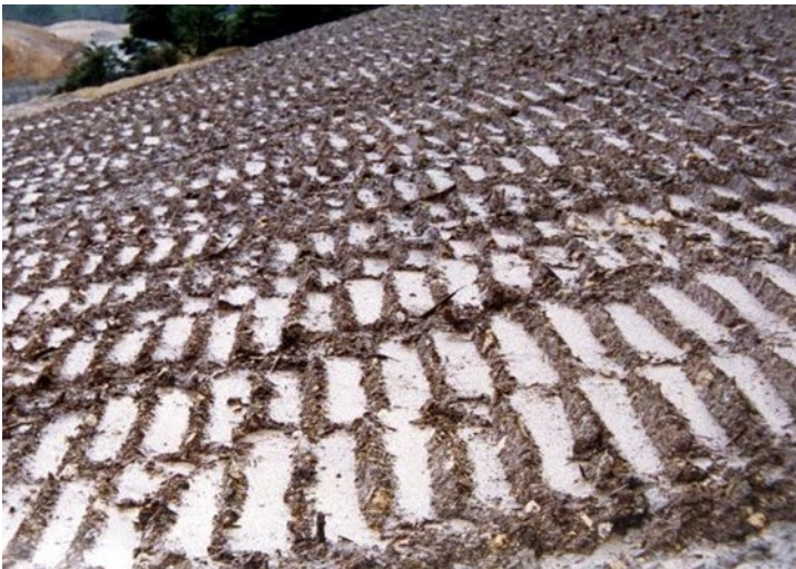
Figure 40: Surface roughening of a slope. Note the hollows acting as "micro" sediment traps
