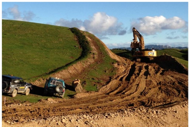
Figure 15: Clean water diversion used to isolate upper clean water flows from the works area
