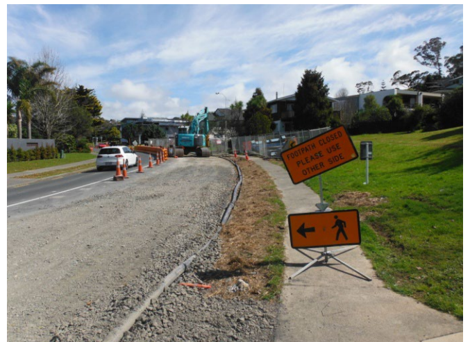
Figure 110: Use of stabilisation products and progressive stabilisation
