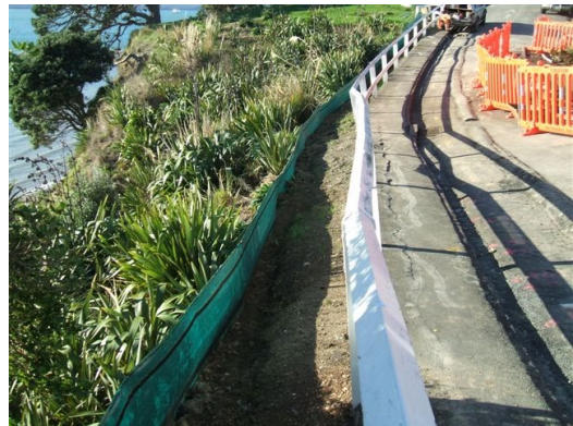
Figure 80: Silt fence installed on edge of works
