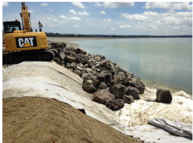
Figure 134: Use of geotextiles and coastal protection rock
