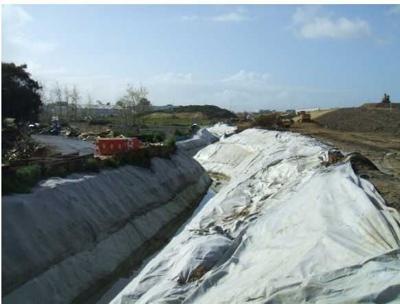
Figure 118: Examples of temporary stream diversion installed to allow permanent culverts to be installed off-line
