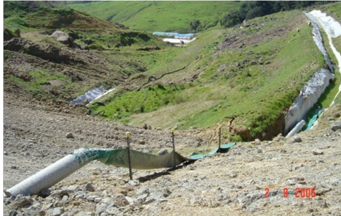
Figure 12: Flume installed to protect steep slope
