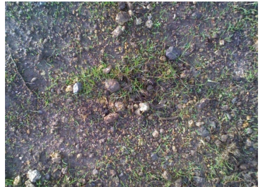
Figure 44: Initial grass strike - not stabilised
