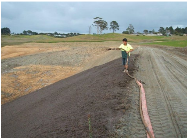
Figure 55: Hydromulch application
