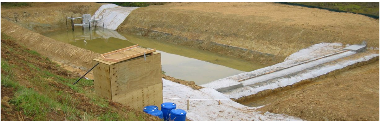
Figure 10: A typical earthworks construction site
