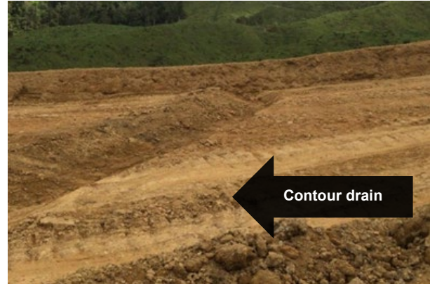
Figure 22: Contour drain
