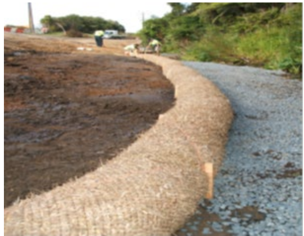
Figure 90: Silt sock used to provide control during final landscaping
