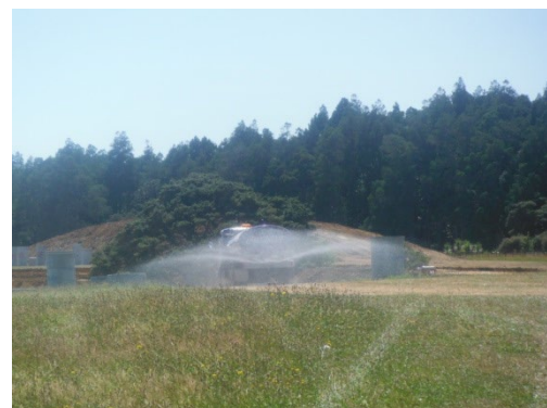
Figure 130: Regular wetting of the haul road
