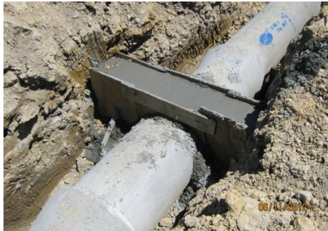
Figure 71: Example of an anti-seep collar
