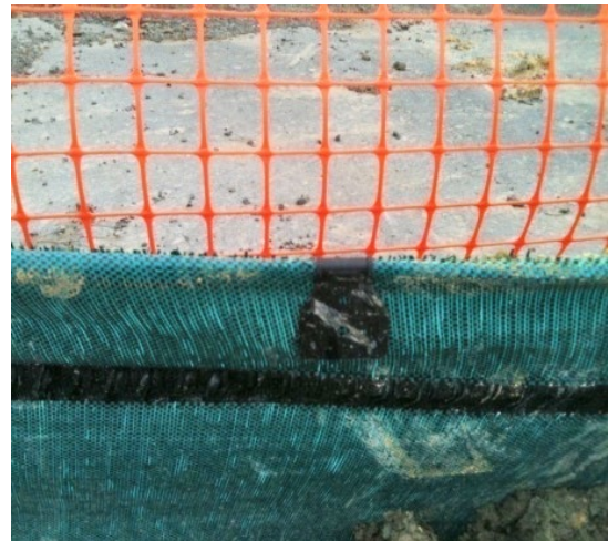
Figure 86: Use of silt fence clips
