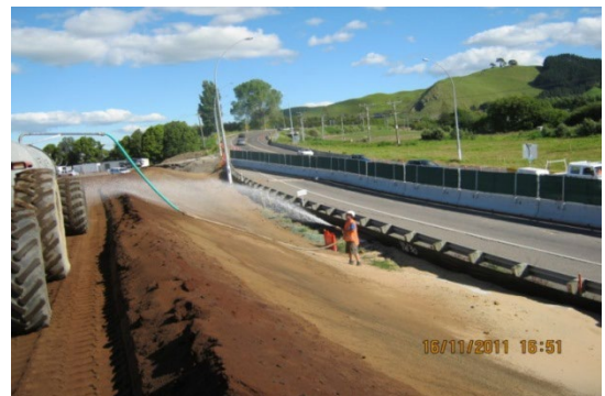
Figure 128: Dust suppression using soil binders/polymers
