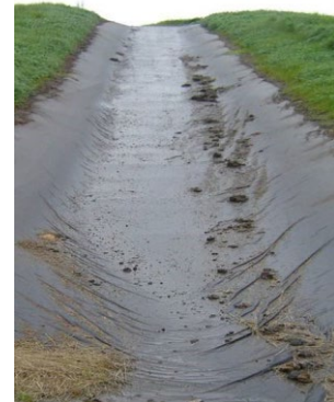
Figure 31: Geotextile lined flume
