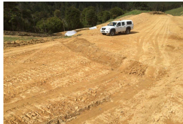
Figure 23: Contour drain installed across access track
