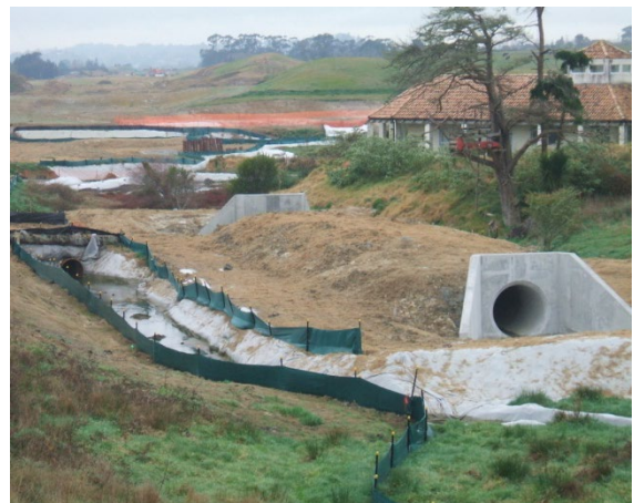
Figure 118: Examples of temporary stream diversion installed to allow permanent culverts to be installed off-line
