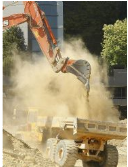
Figure 125: Forward planning and management to minimise dust provide the best options for control
