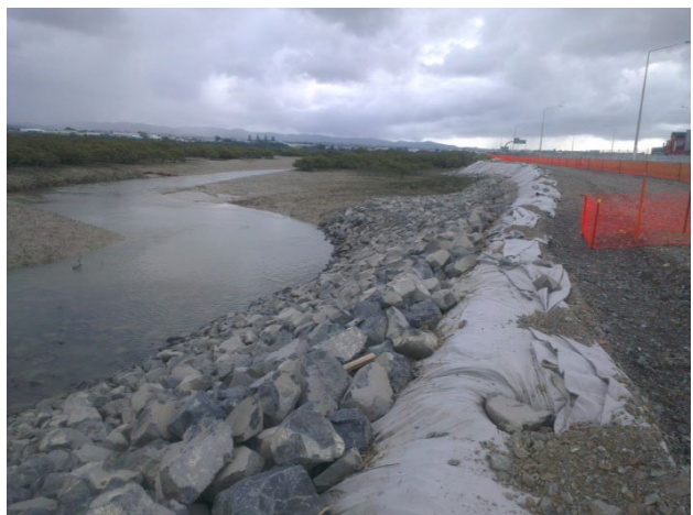
Figure 131: Examples of geotextile filter layer beneath a rock revetment and use of rip rap (SouthernSkies, 2018)
