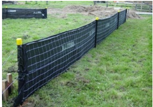
Figure 87: Super silt fence
