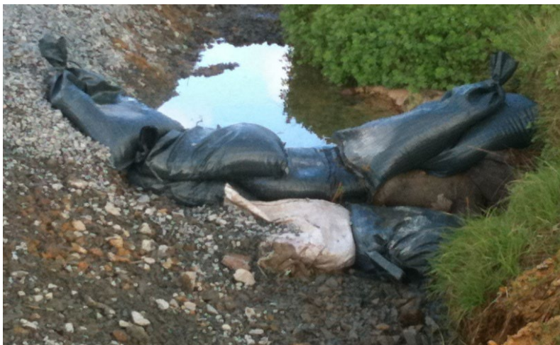
Figure 28: Check dams installed with a spillway to direct flows over the centre of the structure. Sand bags placed directly below spillway provide a protective apron below the dam
