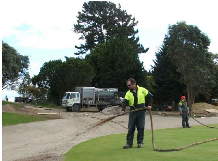
Figure 48: Specialist application of hydroseed
