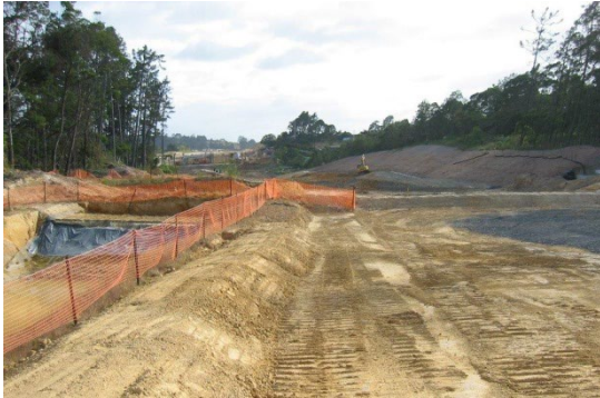
Figure 20: Dirty water diversion bund directing site water to a sediment retention pond
