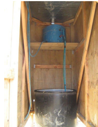
Figure 103: Header tank
