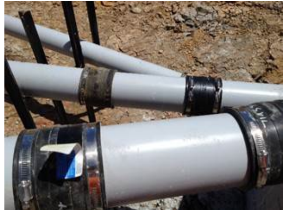
Figure 77: Steel strapping used to attach decant system to horizontal pipework
