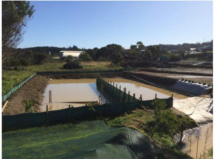
Figure 68: Example of baffles
