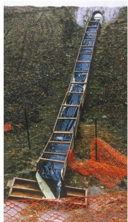
Figure 32: Wooden flume lined with impervious material
