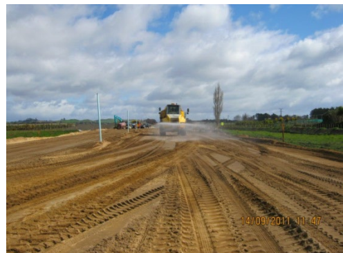
Figure 129: Water truck dampening down the works area
