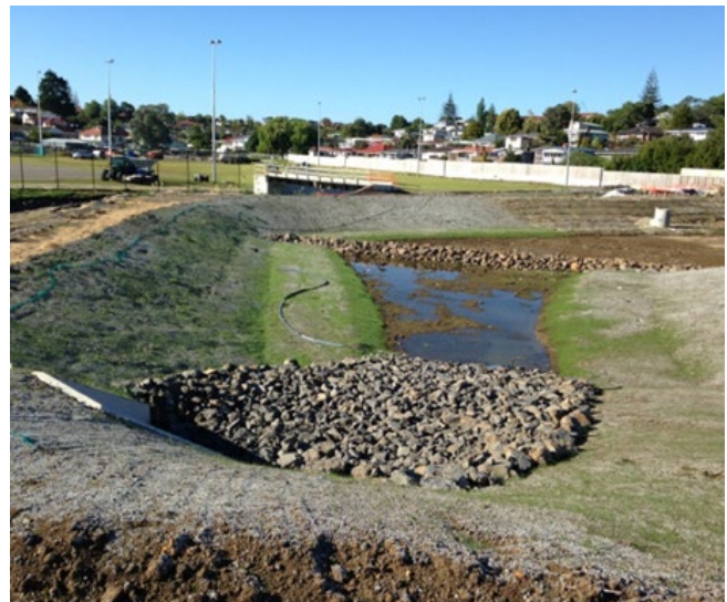
Figure 50: Recently applied hydroseed on a stormwater wetland
