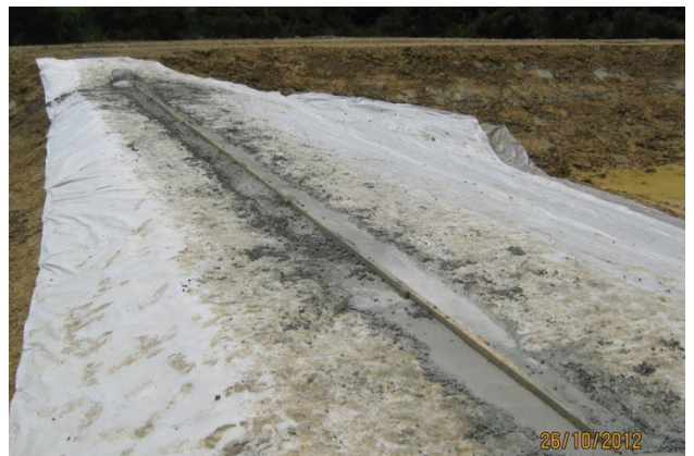
Figure 69: Example of a level spreader
