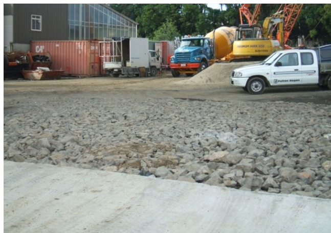
Figure 35: Stabilised entranceway
