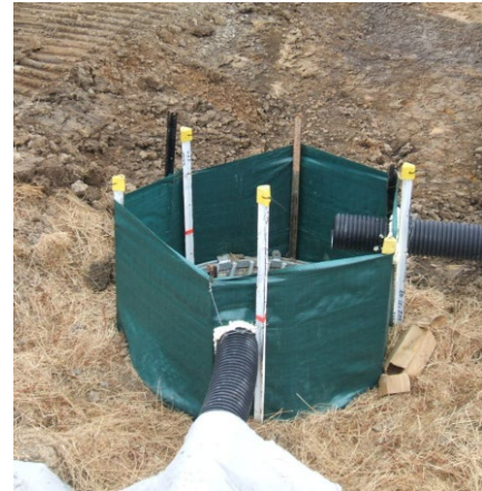
Figure 98: Good use of a silt fence installed to protect a new stormwater catchpit where impounded water will not create a flooding hazard
