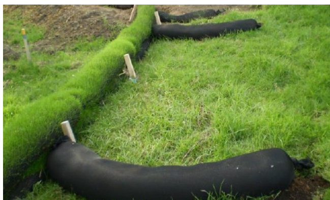
Figure 91: Compost silt socks with returns installed
