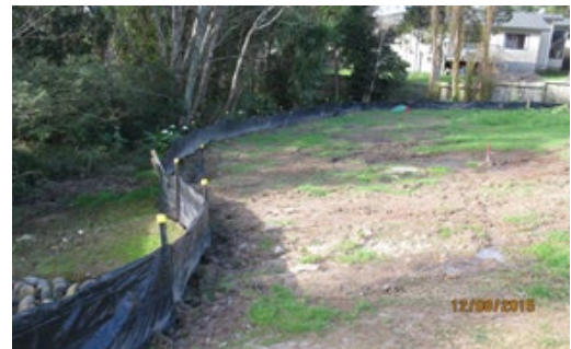
Figure 108: Silt fence
