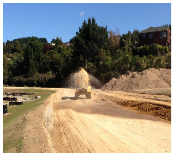
Figure 126: Dust suppression using a water cart
