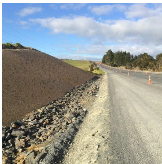
Figure 57: Woodchip to stabilise the finished batter slope
