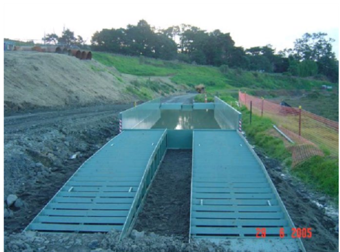
Figure 38: Example of a shaker ramp
