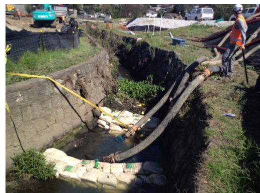
Figure 117: Commencement of over pumping to allow for in-stream works
