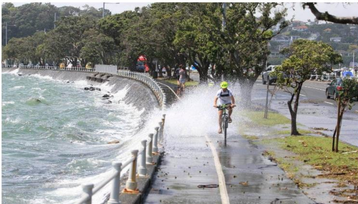
Figure 9: Storm conditions elevating water levels overtops Tamaki Drive Seawall, floods road. (Source: Simon Maude Stuff)
