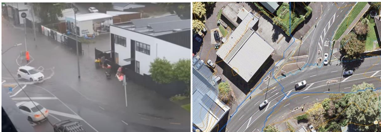
Figure 6: Overland flow path Asquith Avenue, Mt. Albert. The left-hand image is a photo taken of the Asquith Ave / New North Road intersection during an extreme rain event 2023. The right-hand image is an extract from GeoMaps of the same intersection showing the mapped overland flow paths. The blue lines indicate the overland flow path.
