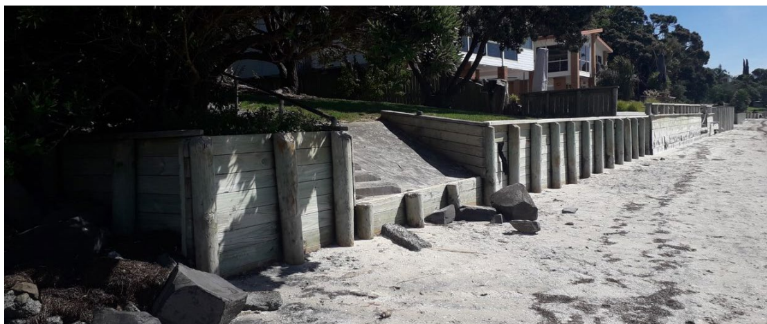
Figure 5-27: Bradleys Access showing timber seawall and access point to the beach
