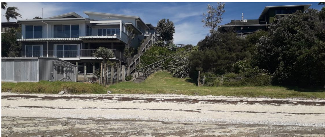
Figure 5-23: Irwins Beach accessway. The sandy beach is backed by a narrow low-lying area of grass reserve established over the stable backshore along the base of the vegetated bank that slopes up to private properties.
