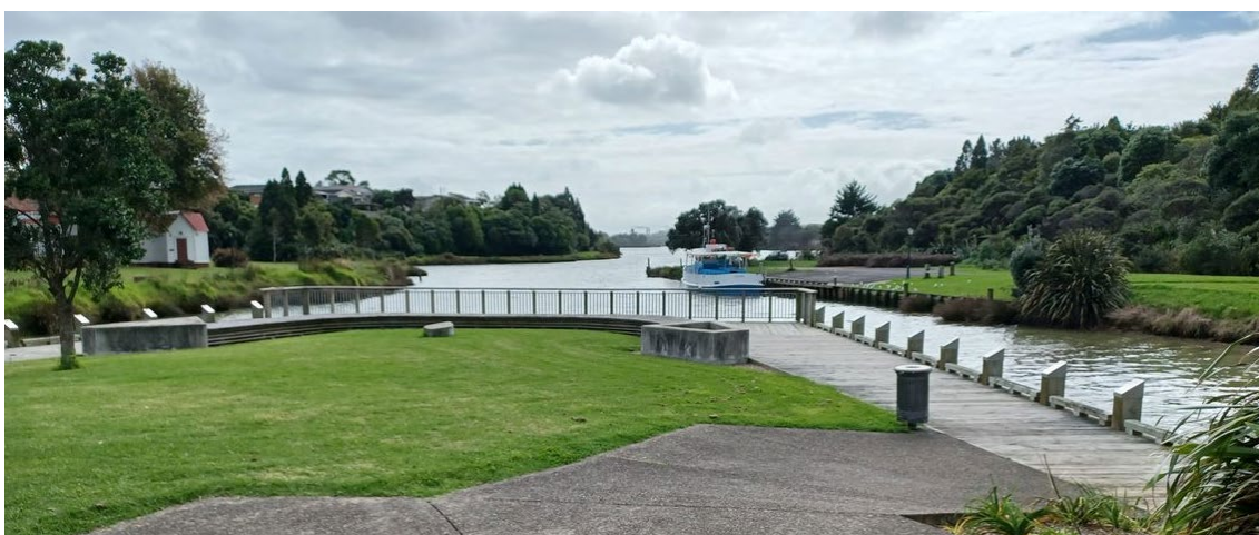
Figure 5-8: Tamakae Wharf in Waiuku Town centre
