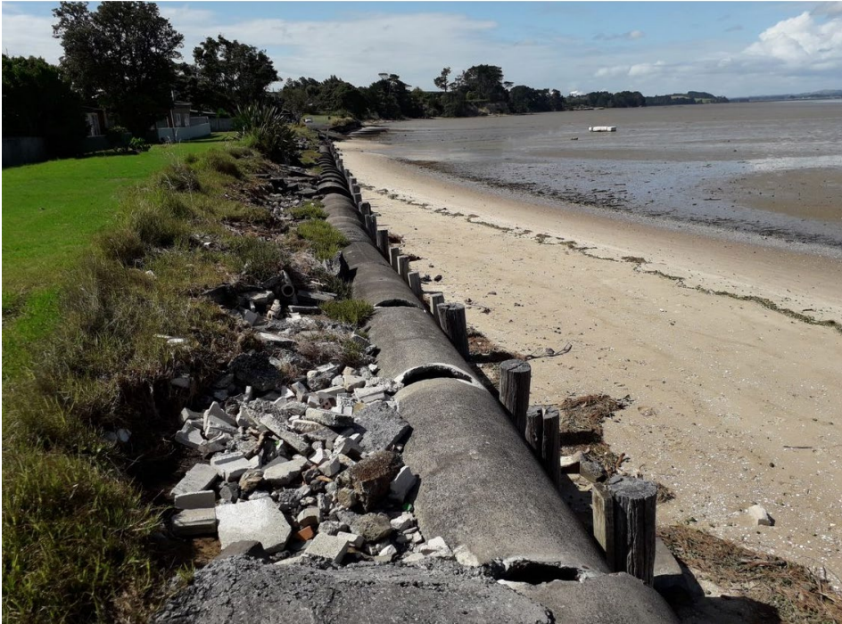
Figure 5-14: Glenbrook beach seawall and beach front
