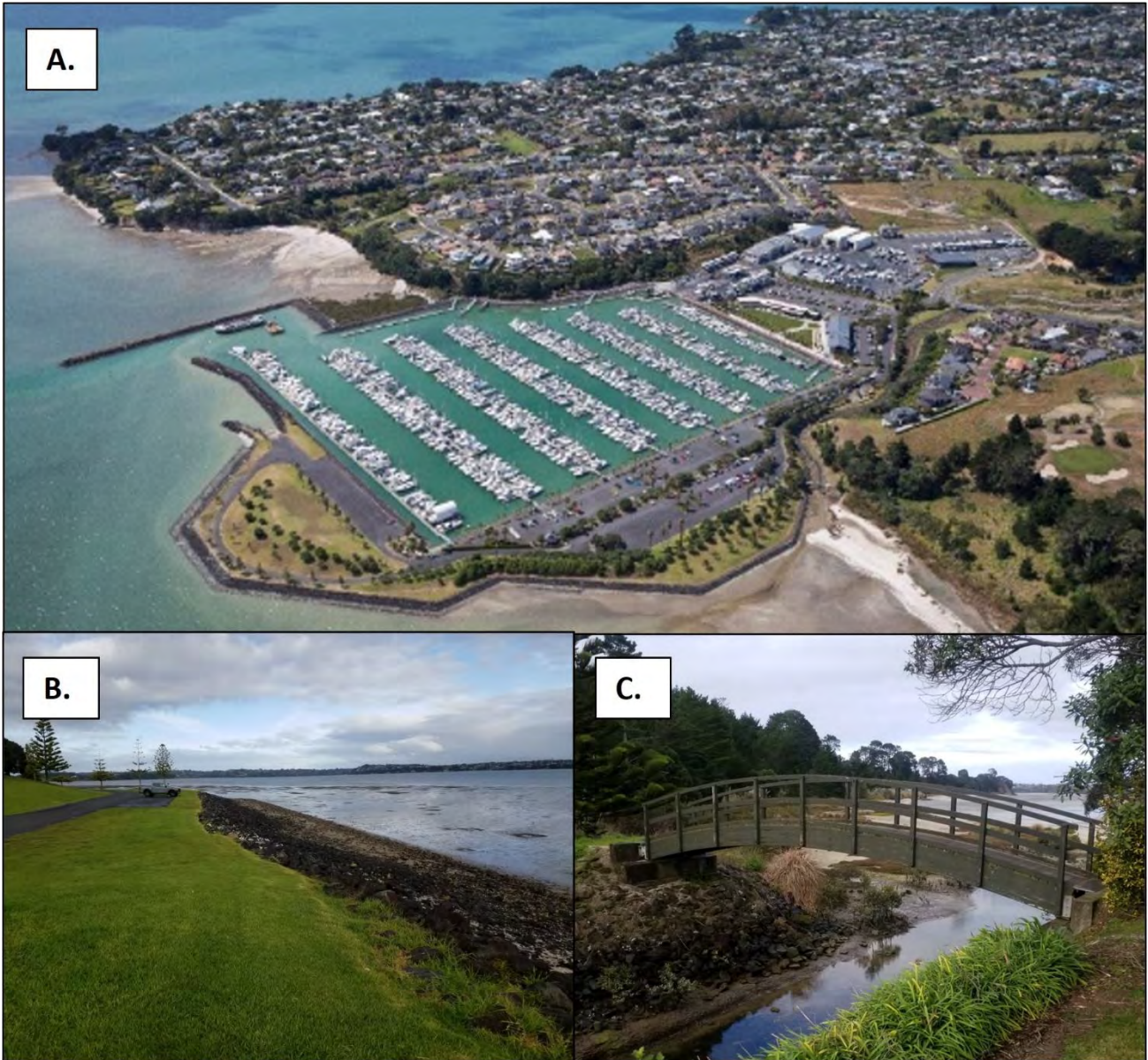
Figure 14 A) Aerial view of Kahawairahi/Pine Harbour marina, B) western revetment (photo facing south), C) pedestrian bridge linking the carpark to Kahawairahi/Pine Harbour Beach
