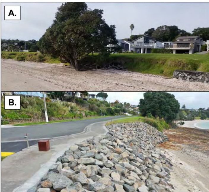
Figure 22: Photo of low-lying cliff edge (A) and the revetment protecting Te Pene Point (B)
