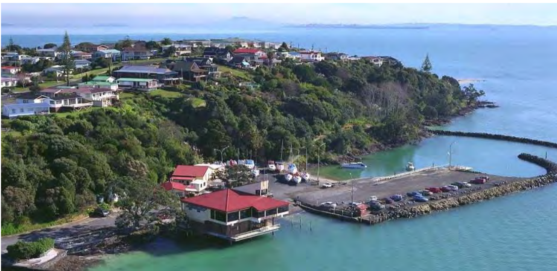
Figure 23: Aerial photograph of Maraetai Boat Club and coastal stretch 10
