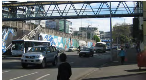
Poor pedestrian experience along route of Fanshawe Street and Hobson Street.
